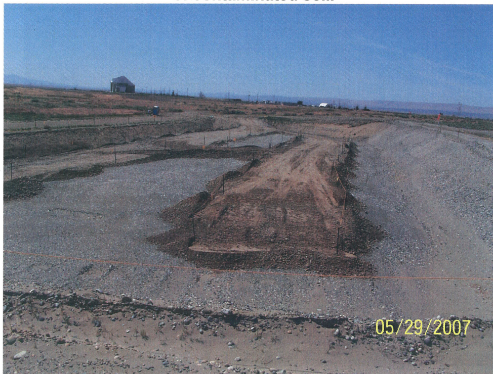
Padding (layer of clean soil) installed to minimize spread of contamination during continued excavation and load-out of contaminated soil.
