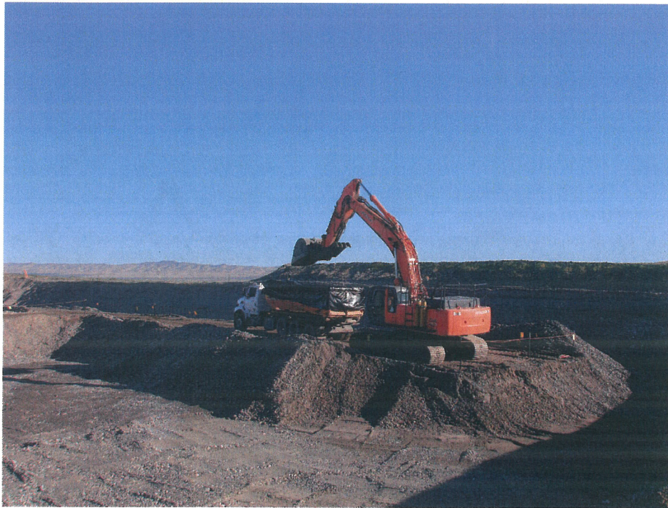
118-F-5 Burial Ground excavation being backfilled (September 2007).
