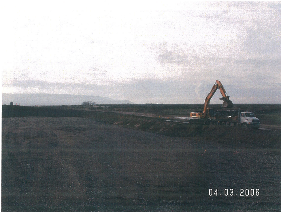
Padding (layer of clean soil) installed to minimize spread of contamination during continued excavation and load-out of contaminated soil.
