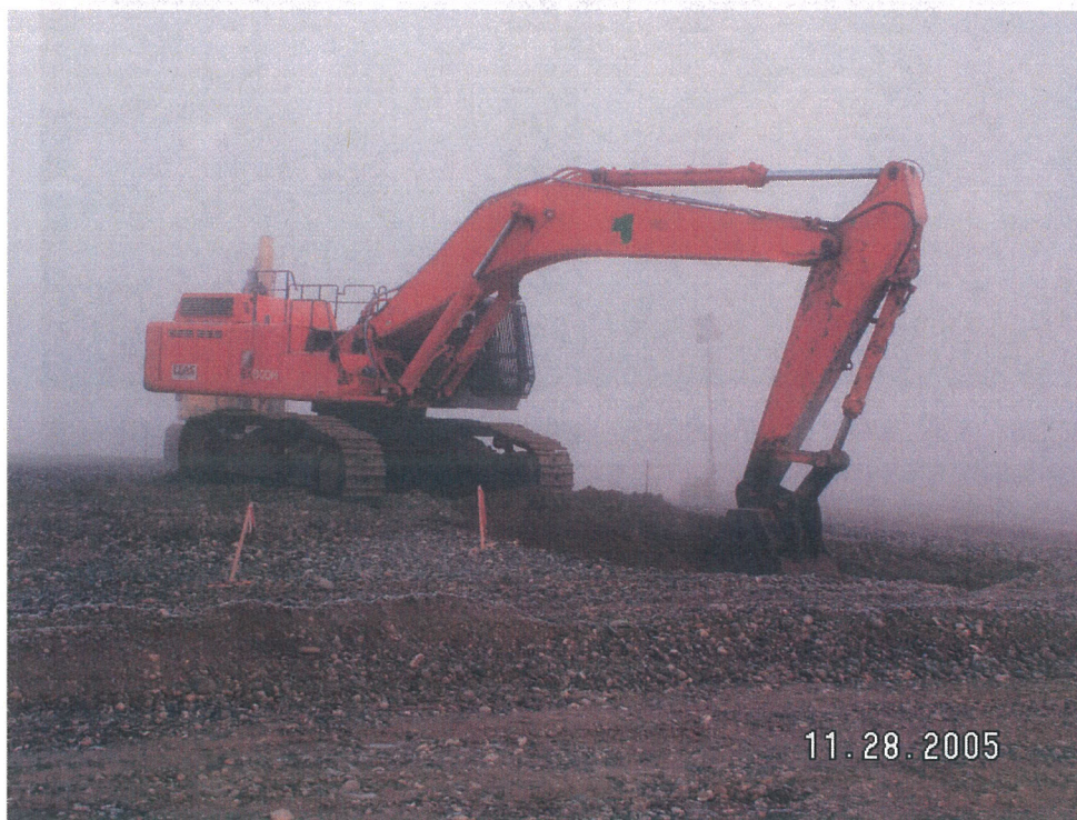
Removal of overburden at 118-F-5 Burial Ground.
