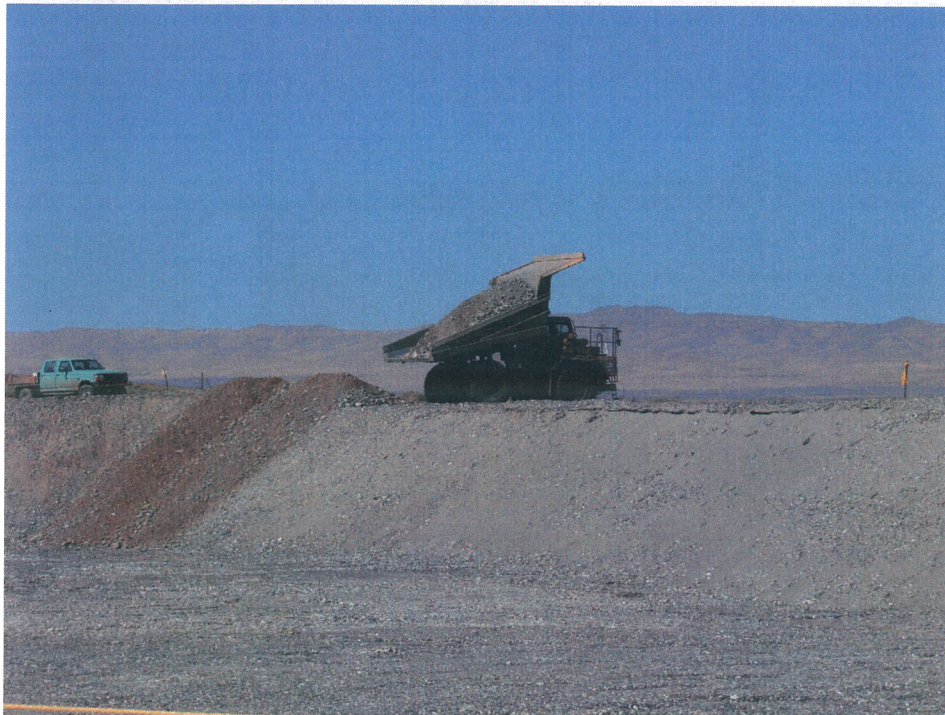
118-F-5 Burial Ground excavation being backfilled (September 2007).
