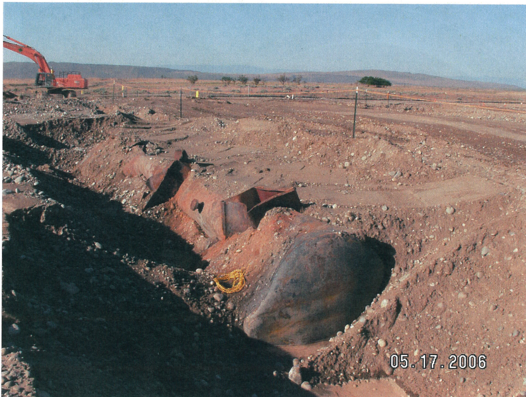
Railroad Tank Car in Trench 6 with Manhole Visible.
