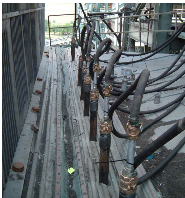
Figure 6.1-5 Sorbent Injection Lances
