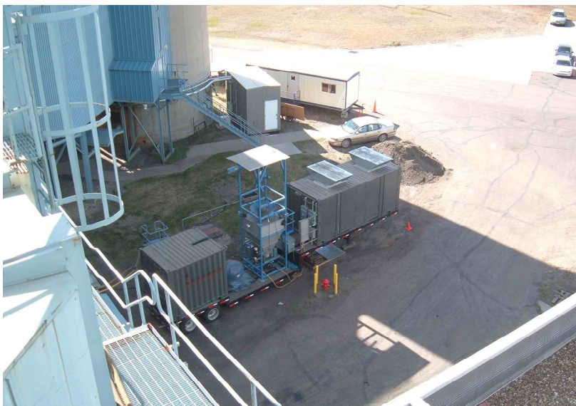
Figure 6.2-5 Mer-Cure™ System After Installation
