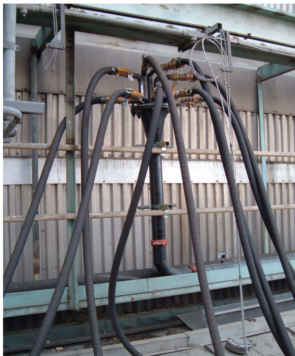
Figure 6.1-4 Sorbent Distribution System
