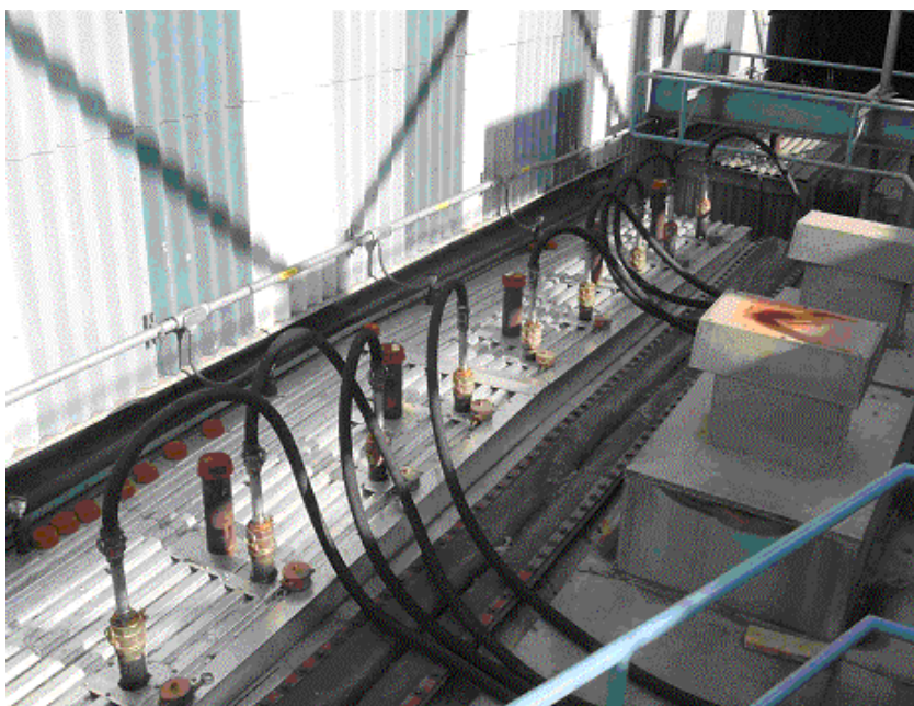
Figure 6.2-4 Sorbent Injection Lances Installed Upstream of the Air Heater
