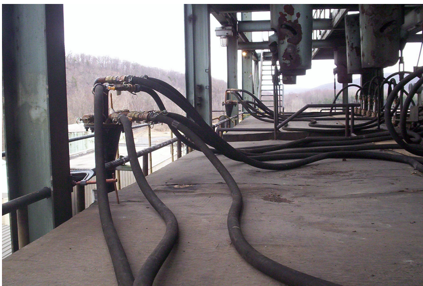
Figure 6.3-3 Sorbent Distribution and Injection System at the Economizer Outlet
