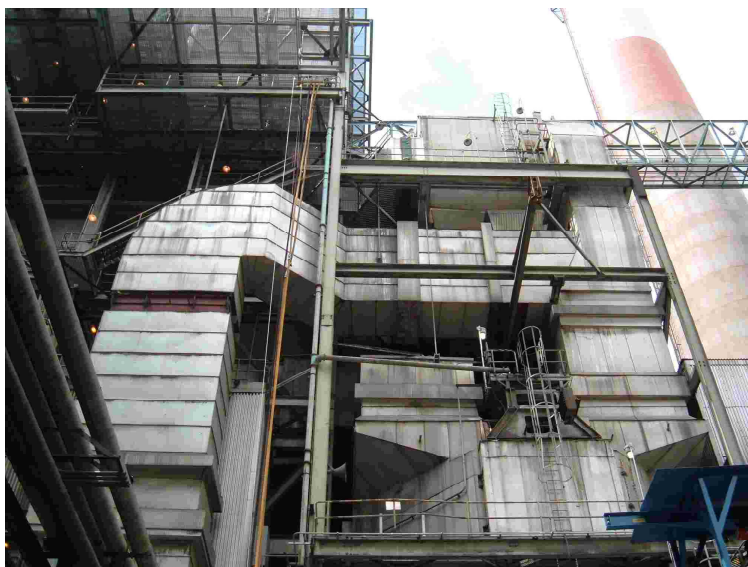
Figure 6.1-1 Sorbent Injection Between Economizer and Air Heater for Dave Johnston Unit #3
