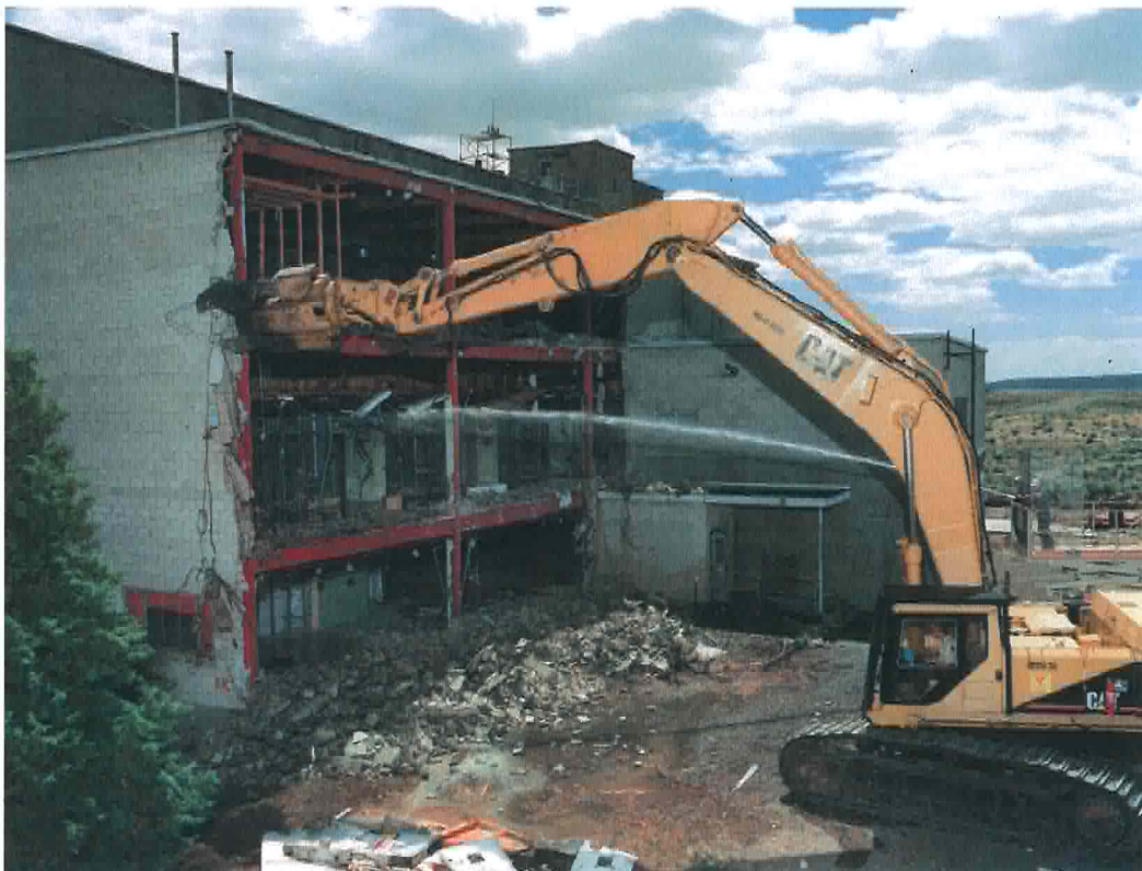
Photograph A-2. Heavy Equipment Removing Concrete Wall on West Side of 108-F Biological Laboratory as Water is Sprayed to Control Dust (1999).
