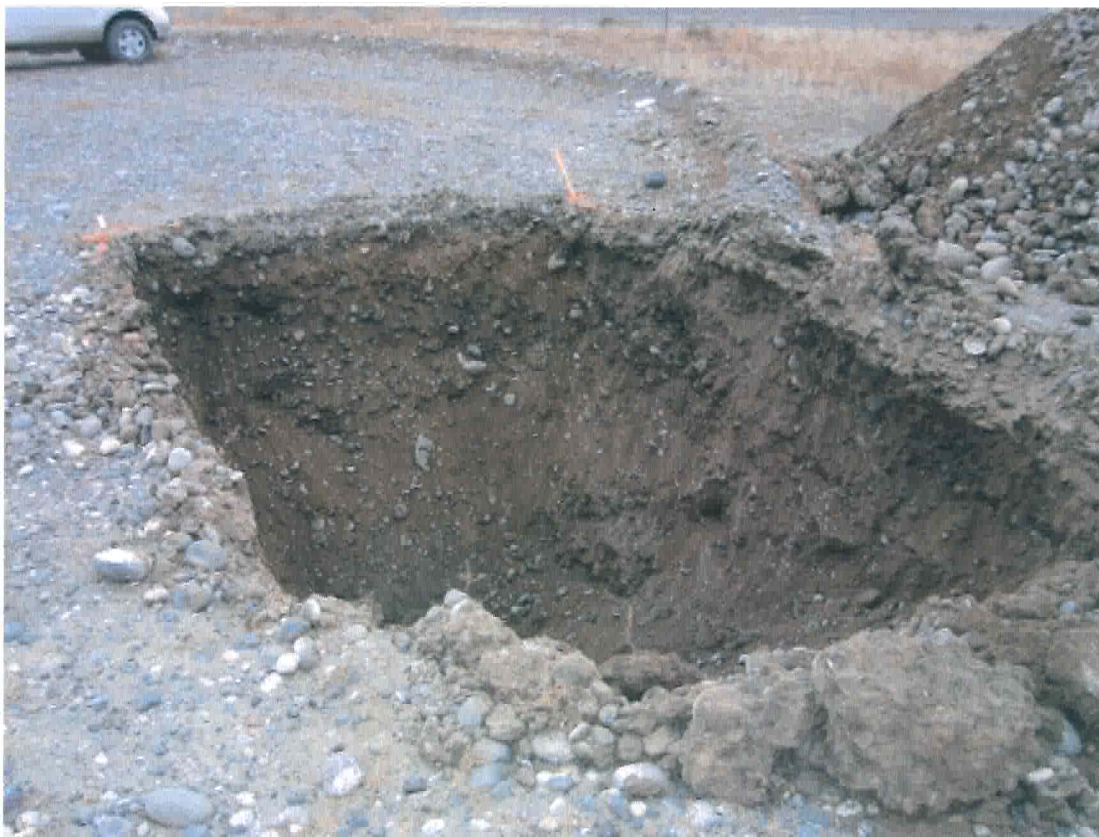
Photograph A-6. Excavation of Test Pit 1 for Sampling (December 2006).
