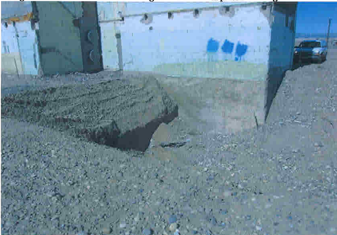
Figure 9. 105-F Reactor Building Foundation Exposed During Excavation.
