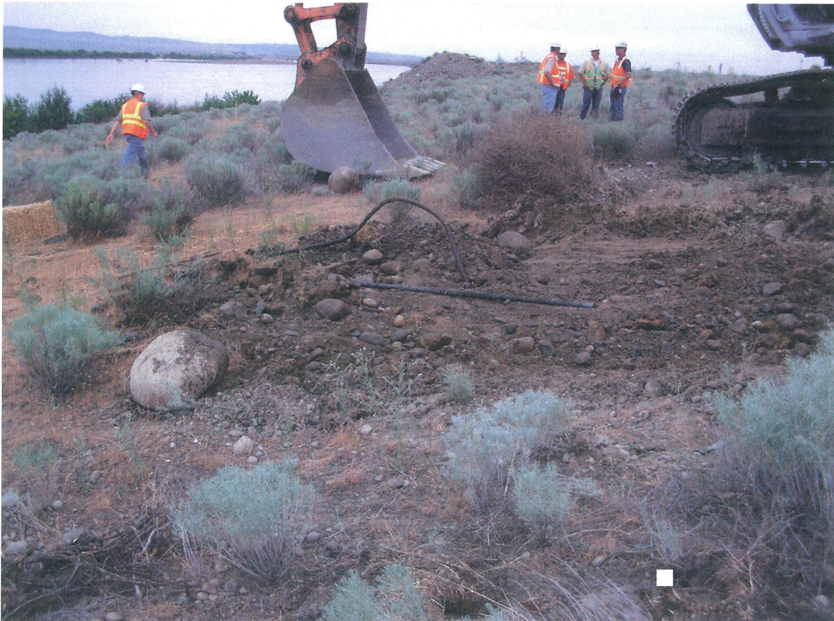
Figure 3. Remediation of the 100-B-21:2 Waste Site.
