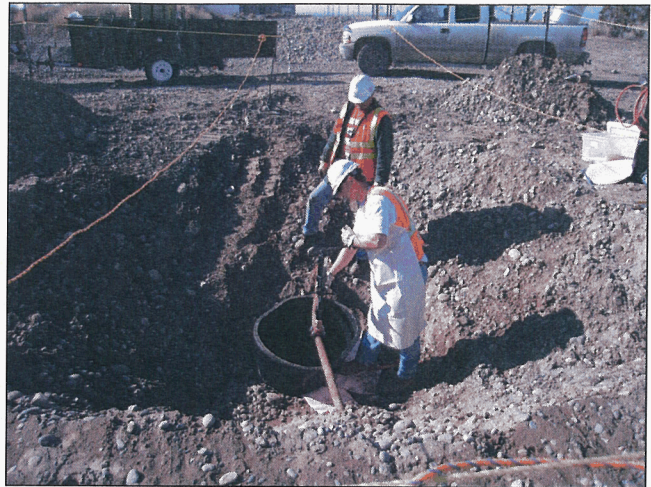
Allowing Hot Tap to Drain.
