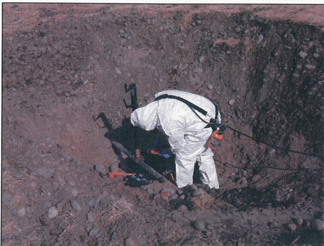
Dis-assembling Hot Tap in Level B PPE.
