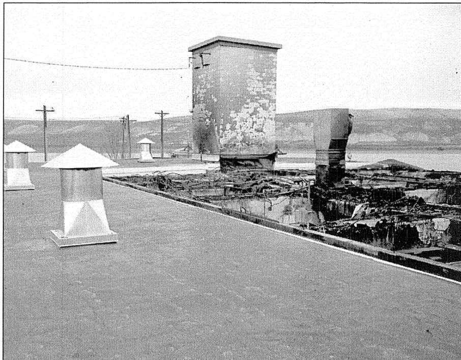
146-FR Laboratory. Another View of Burned Roof of Facility.
