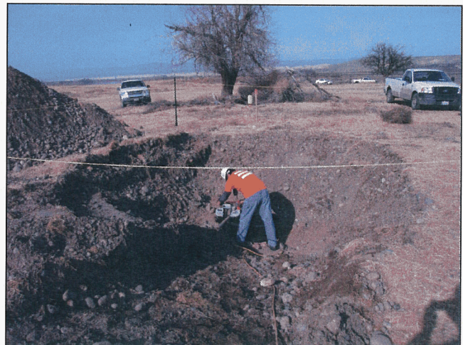
Cutting Open Pipe Using Band Saw.
