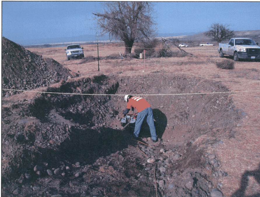
Figure 11. Cutting Open Pipe with Band Saw at 100-F-52.
