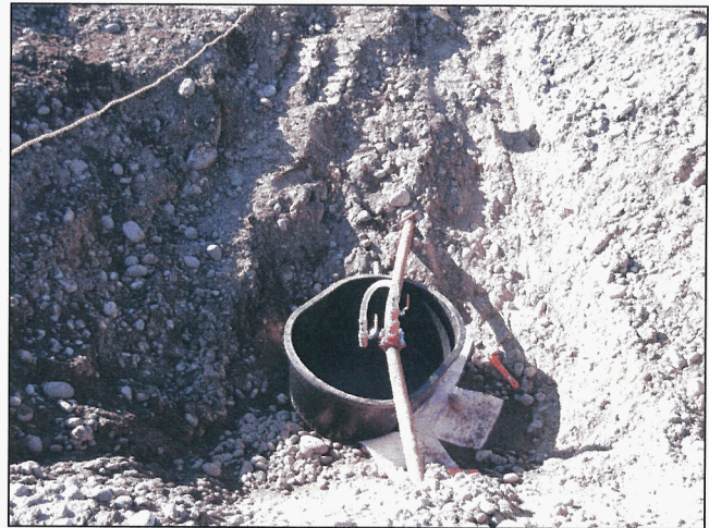
Cutting Open Pipe Using Band Saw.
