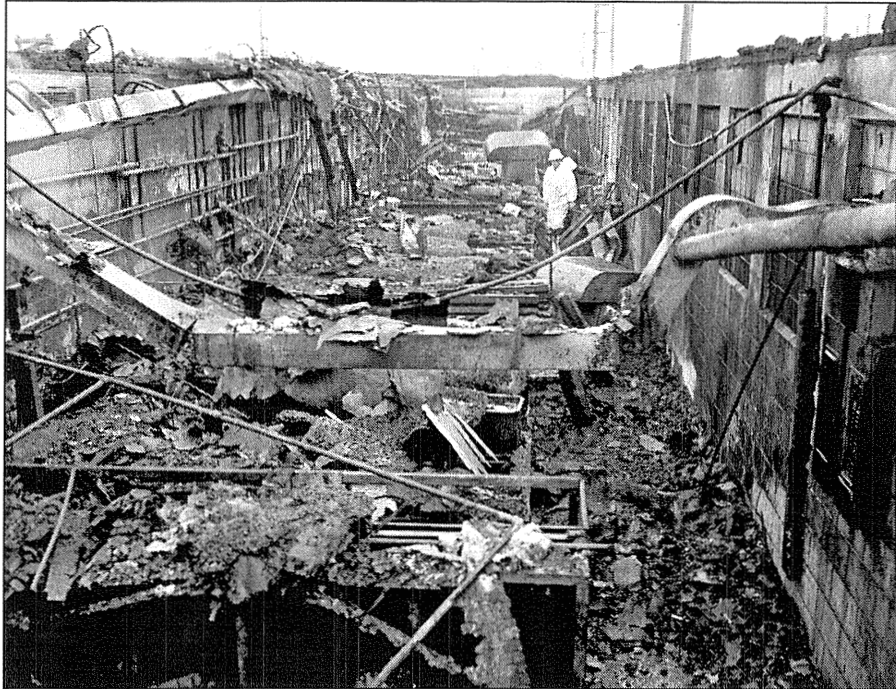
146-FR Laboratory. Another View of Burned Roof of Facility.
