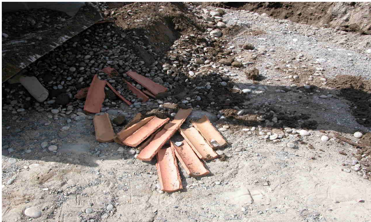
Photograph B-3. Clean Interior of Vitrified Clay Pipe Laterals in the 331 LSLDF.
