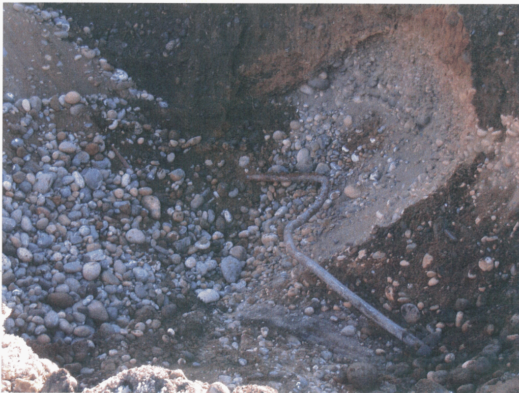
Close-Up View of 0.05 m (2-in.) Steel Pipeline (January 16, 2008).
