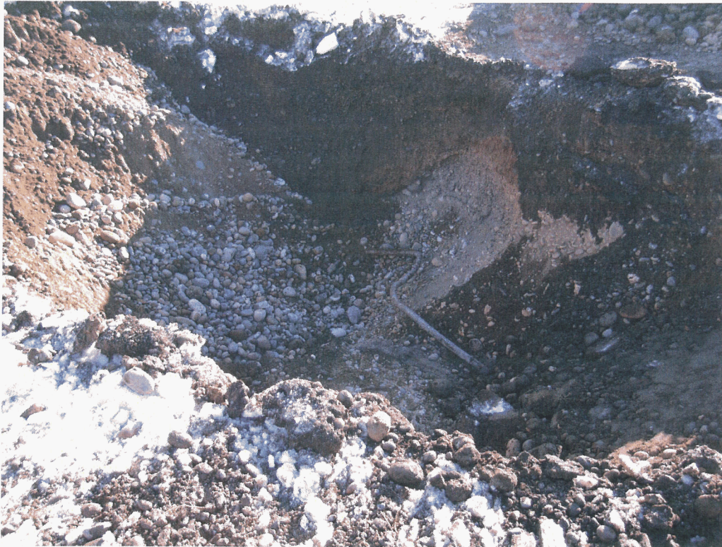
Close-Up View of 0.05 m (2-in.) Steel Pipeline (January 16, 2008).
