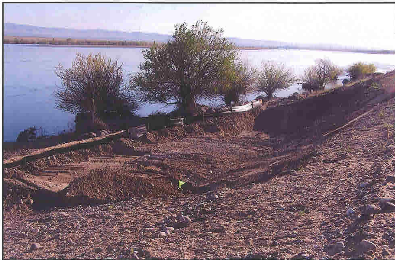
Photograph 7. 128-B-3 River Embankment Area Following Remediation (May 2006).
