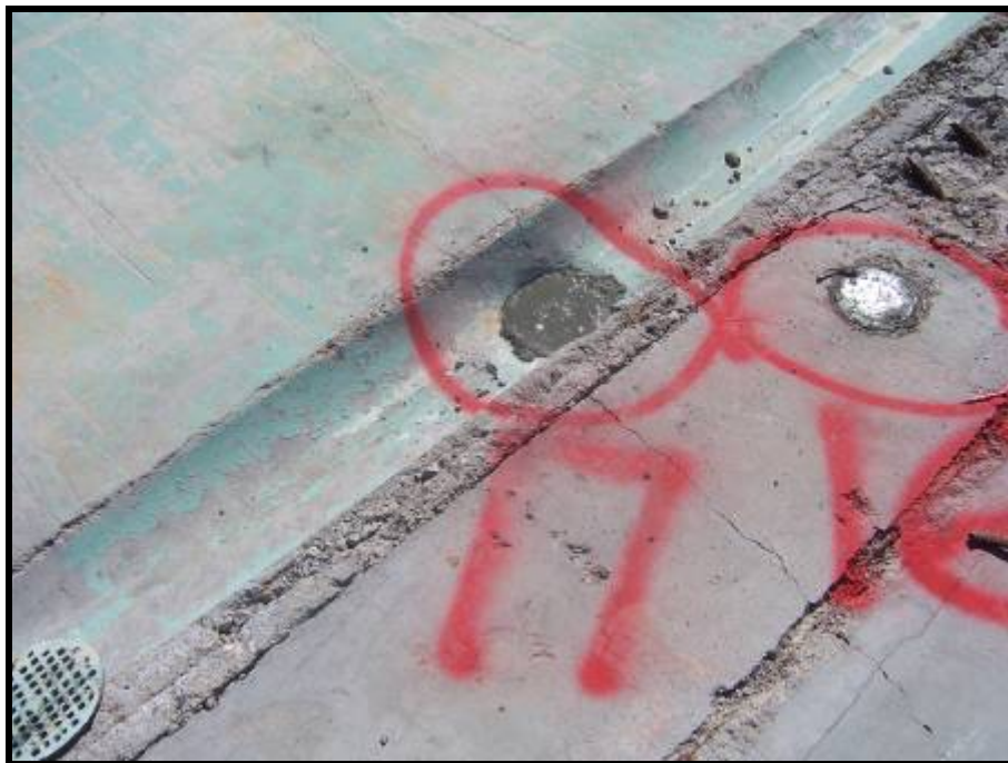
Figure 8. CP-2 Floor Drains Grouted
