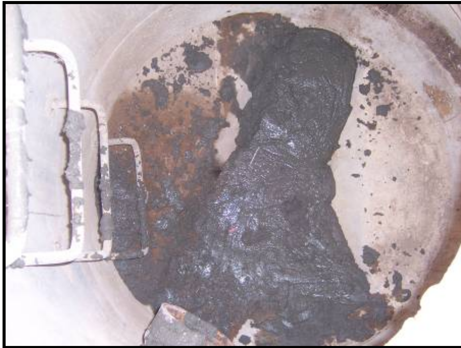
Figure 7. CAS 06-03-01 South Lagoon Manhole Grouted
