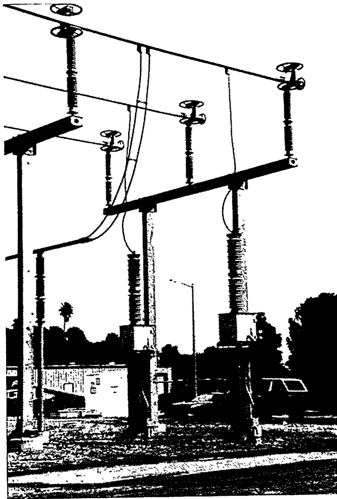
Figure 18. Close-up of typical rigid buswork suspended by short chains. This photo was taken after temporary repairs were made.
