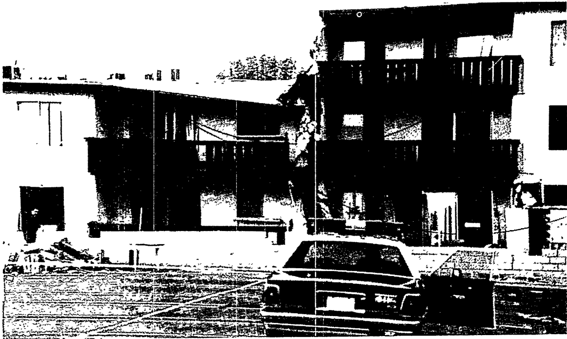
Figure 6. Northridge Meadows Apartments was an example of multi-story apartment buildings built with minimal seismic design details and poor construction practices. Due to collapse of the first story, 15 people were killed at this one apartment complex.
