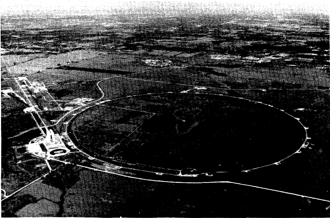
Figure 1-6. Aerial view of the Fermilab accelerator complex. The large circle outlines the underground main ring. The smaller circle at the left is the booster synchrotron, fed by a linear accelerator. The high-rise laboratory building is behind the linac-booster area.
