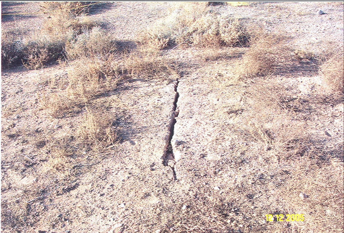
11. Reoccurring subsidence crack on the cover.
