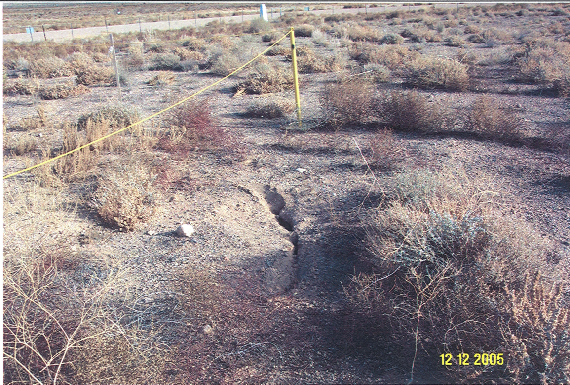
9. Subsidence crack along eastside of the cover.
