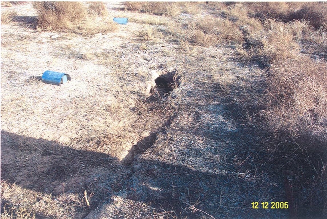
12. Small animal burrow on a subsidence crack.
