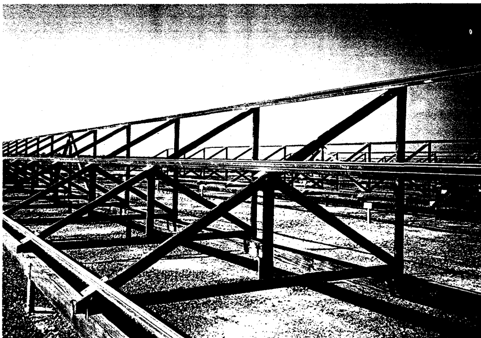
Figure 6-7 Treated Wood Support Structure for EMT-2
