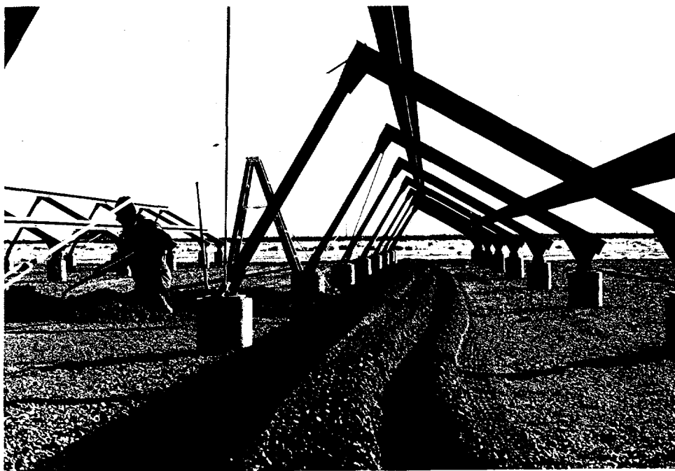
Figure 6-6 Cable-Braced Steel Support Structure for EMT-1
