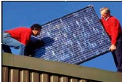
Installing a PV array on a building
