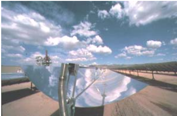
Figure 6-8: Solar Thermal Power Plants- Mojave Desert
