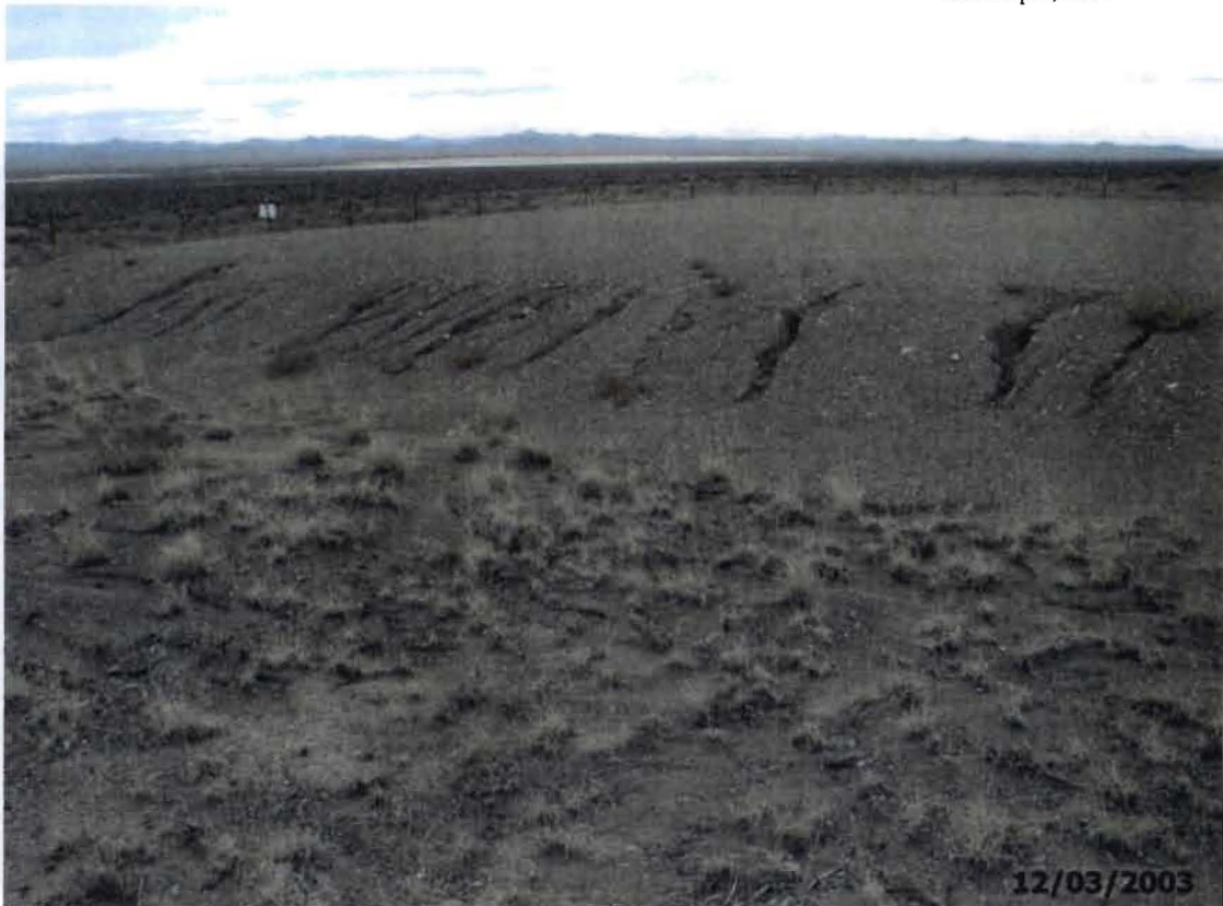
9. CAU 407 Roller Coaster RadSafe Area, looking south showing erosion on cover
