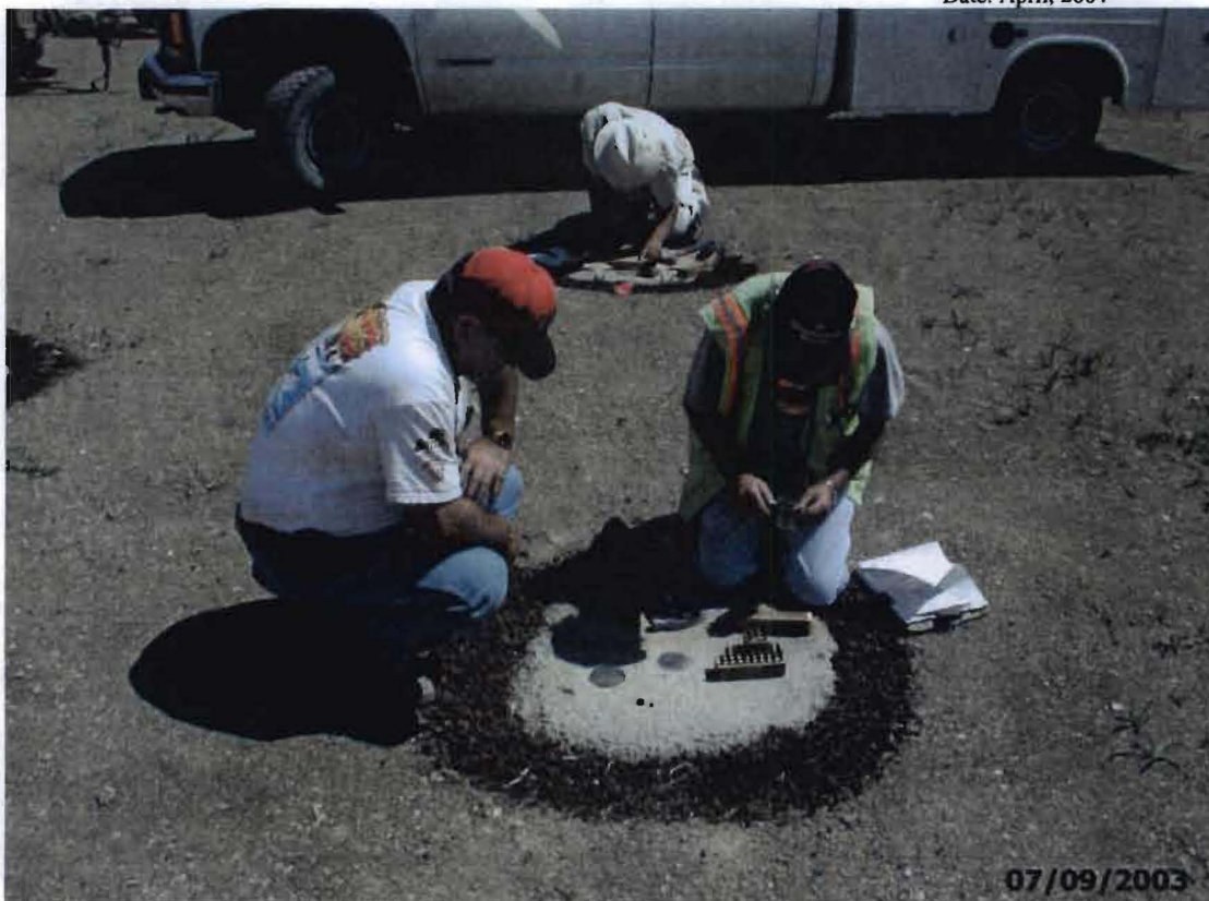
29. CAU 424 Area 3 Landfill Complexes Landfill Cell A3-3, July 2003 repairs (stamping land-use restriction coordinates on monument)
