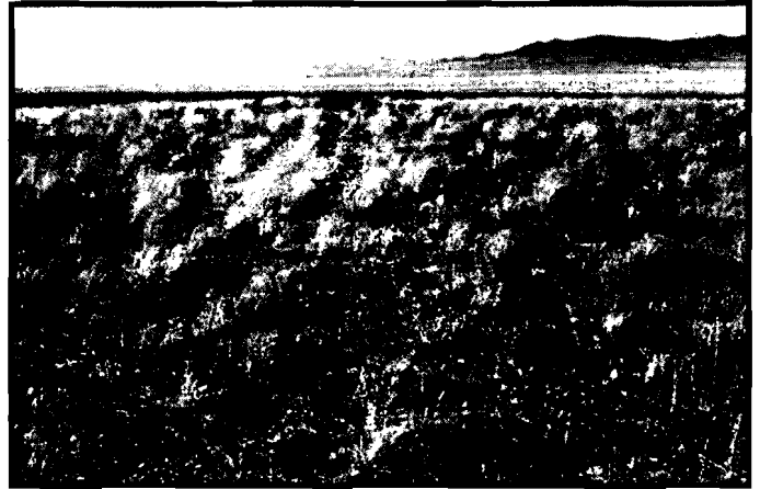
Roller Coaster Sewage Lagoons cover cap photo reference point, June 2000, three years after revegetation. Grasses and shrubs are becoming well established on cover cap. Shrubs are smaller in height and width than those found on the staging area, but shrub vigor is very good.
