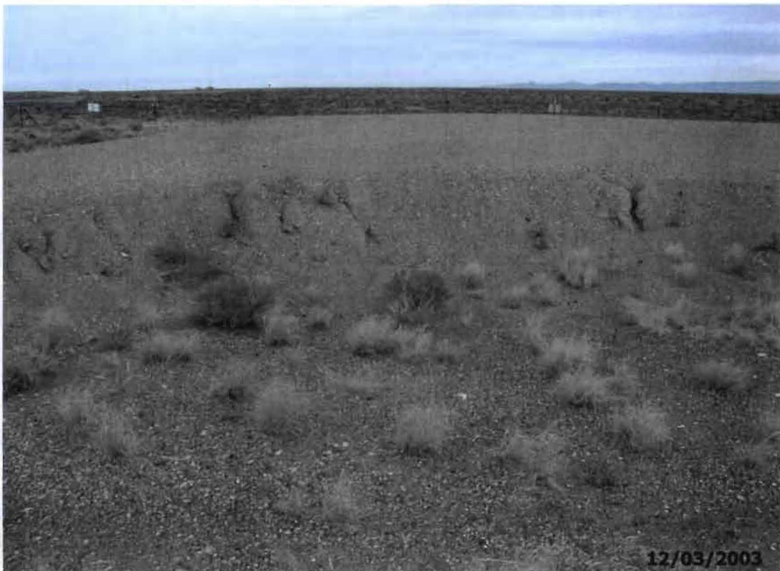
10. CAU 407 Roller Coaster RadSafe Area, looking north showing erosion on cover
