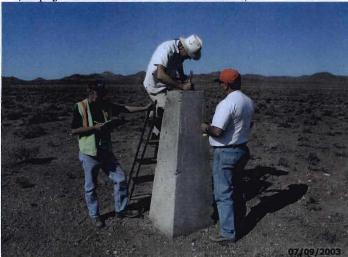
30. CAU 424 Area 3 Landfill Complexes Landfill Cell A3-4, July 2003 repairs (stamping land-use restriction coordinates on monument)
