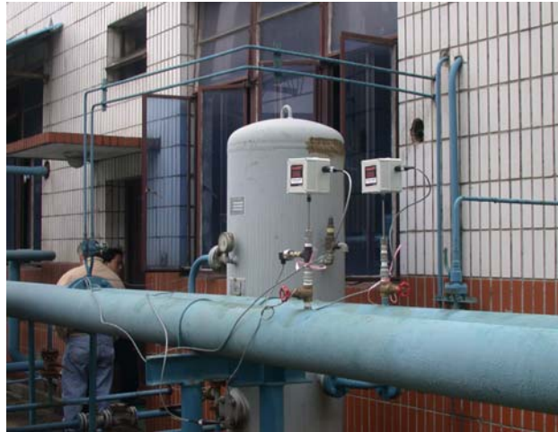
Figure 2 flow measurement with insertion-type mass flow meter
