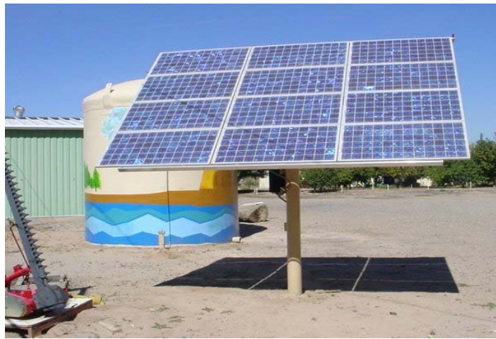
Figure 3. Polycrystalline 1.2 kW PV water pumping system with active tracker, and 10,000 gallon storage tank located at SIPI greenhouse complex. Pumps water for the arboretum, garden, and fruit orchard.
