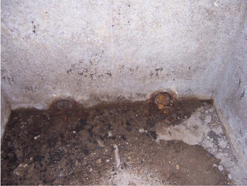
Photograph 25: CAS 12-04-01, System #4, Interior of Distribution Box before Grouting, 03/18/2008
