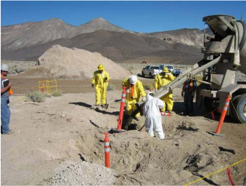
Photograph 7: CAS 12-04-02, Filling Septic Tanks with Grout, 11/20/2007
