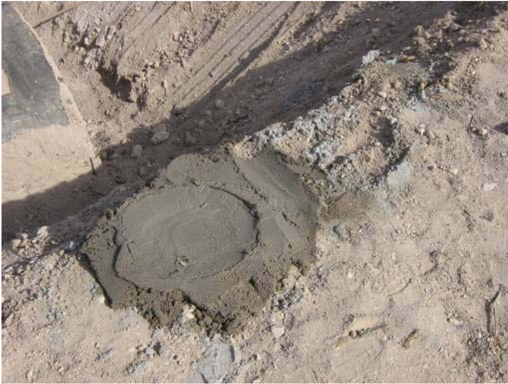
Photograph 13: Remaining Sewage Lines in Area 12 Grouted, 11/28/2007
