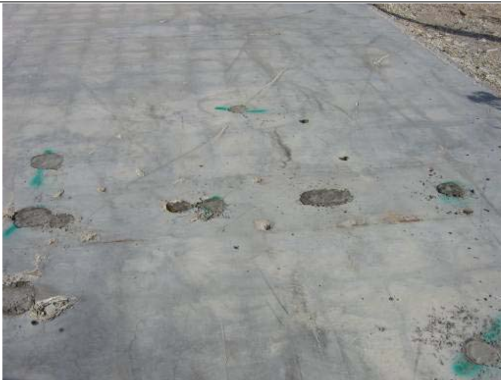
Photograph 11: Sewage Lines on Adjacent Concrete Pad in Area 12 Grouted, 11/28/2007
