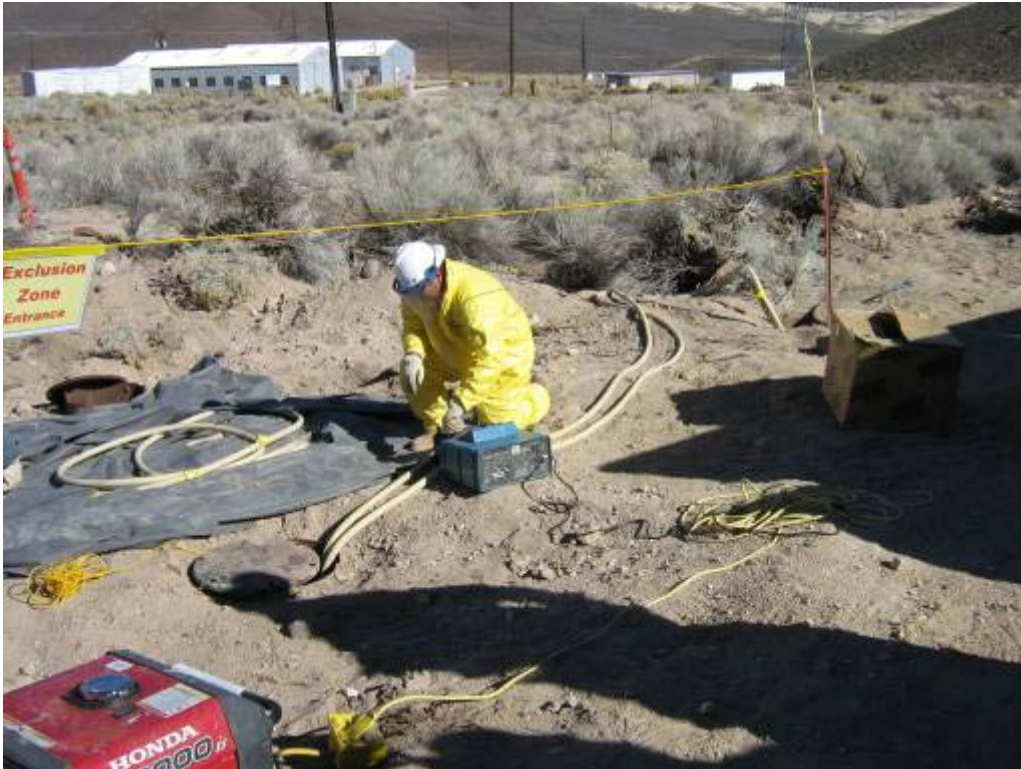
Photograph 6: CAS 12-04-01, Pumping Liquid from System #1 Septic Tanks, 11/20/2007
