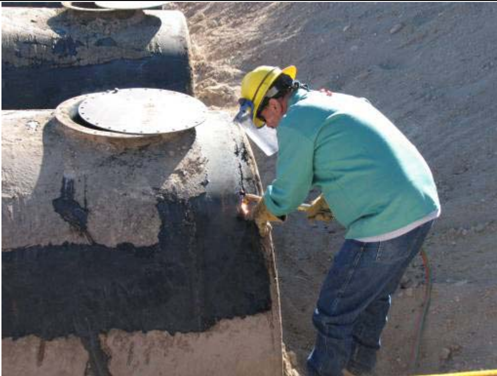
Photograph 9: CAS 12-04-01, Cutting System #4 Septic Tanks, 11/26/2007
