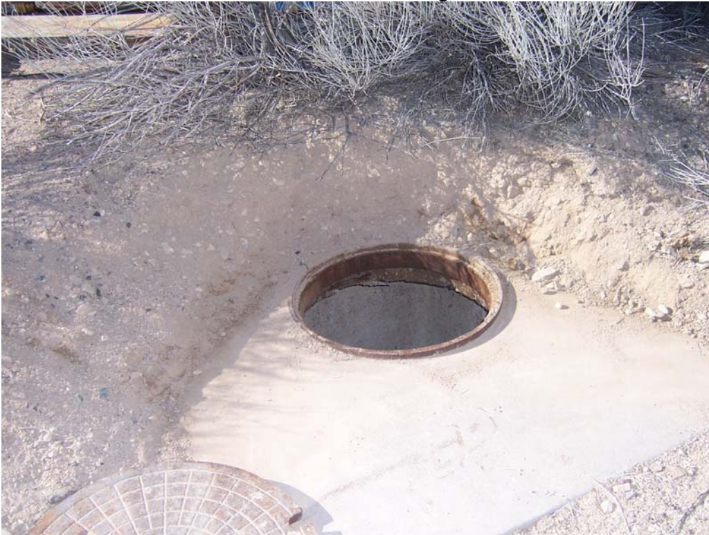
Photograph 26: CAS 12-04-01, System #4, Exterior of Distribution Box before Grouting, 03/18/2008
