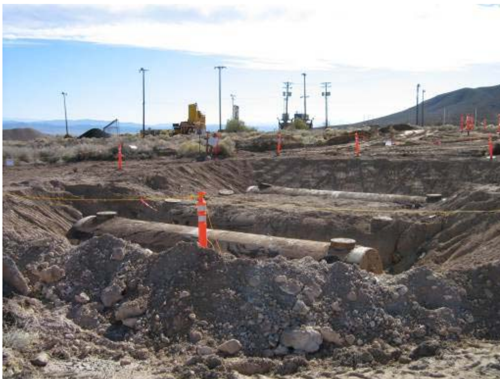
Photograph 4: CAS 12-04-03, Septic Tanks Uncovered, 11/20/2007
