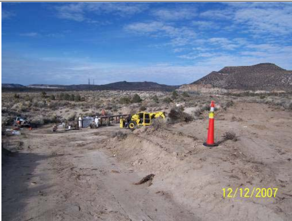
Photograph 19: CAS 18-03-01, Removal of Asbestos Cement Pipe, 12/12/2007
