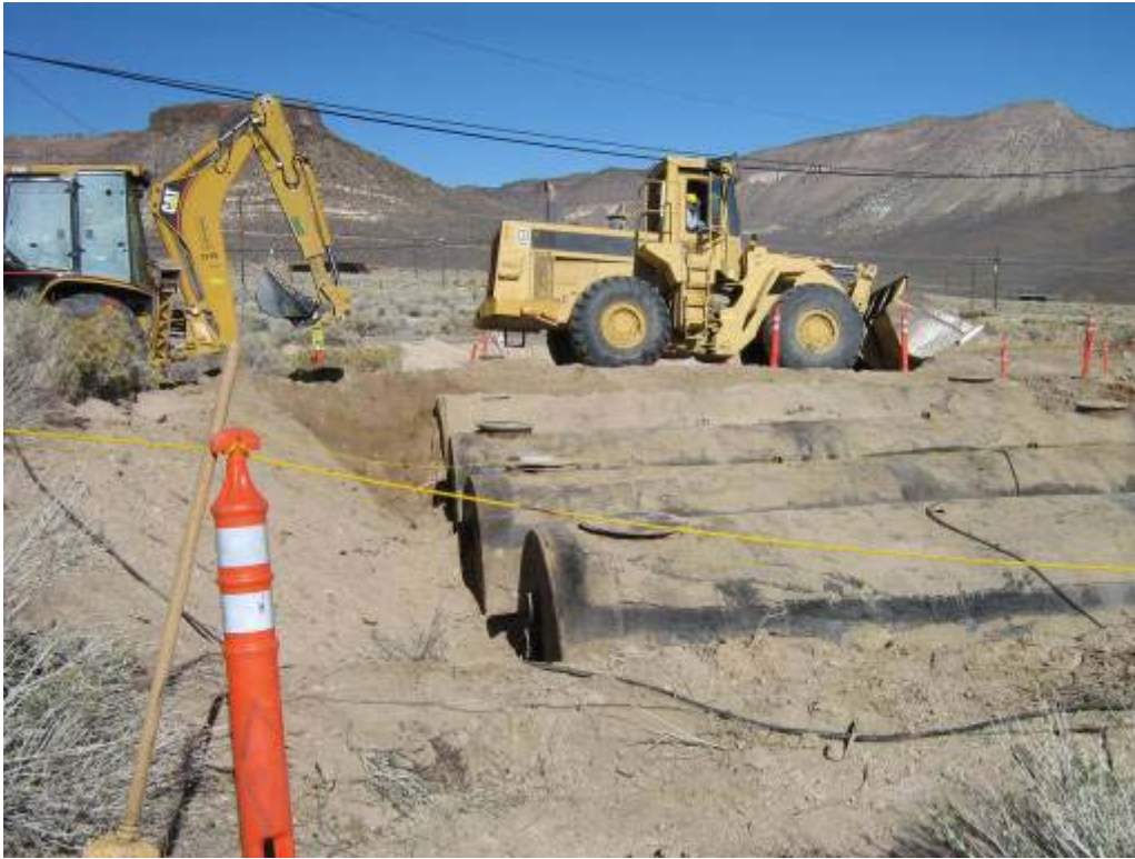
Photograph 5: CAS 12-04-01, System #4 Septic Tanks Uncovered, 11/20/2007
