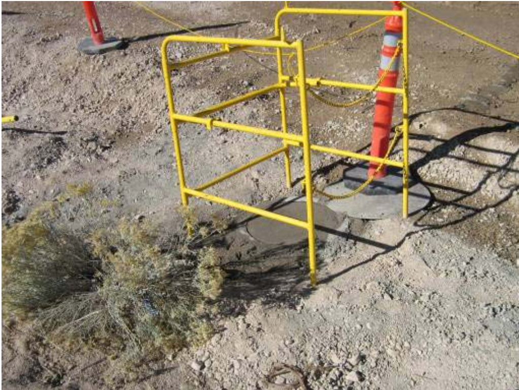
Photograph 8: CAS 12-04-02, Septic Tank Filled with Grout, 11/20/2007
