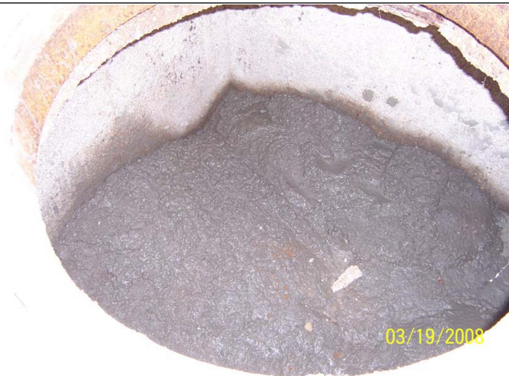
Photograph 27: CAS 12-04-01, System #4, Distribution Box during Grouting, 03/19/2008
