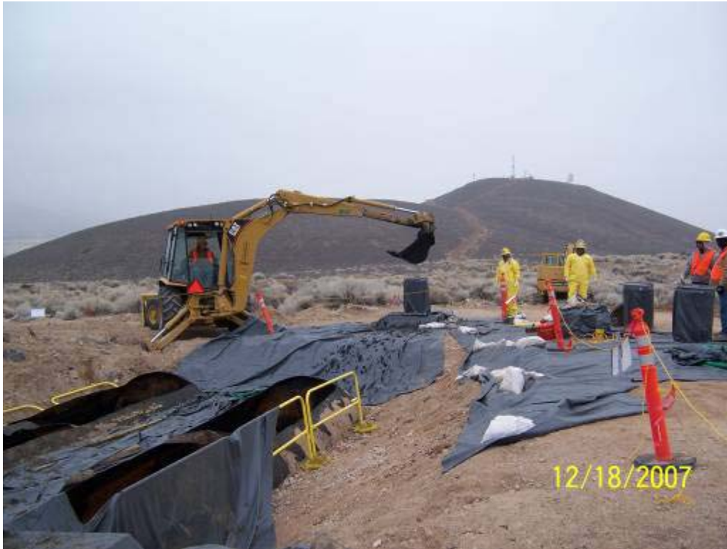
Photograph 21: CAS 12-04-01, Packaging Mixed Waste Sludge from System #1 Septic Tanks into Drums, 12/18/2007
