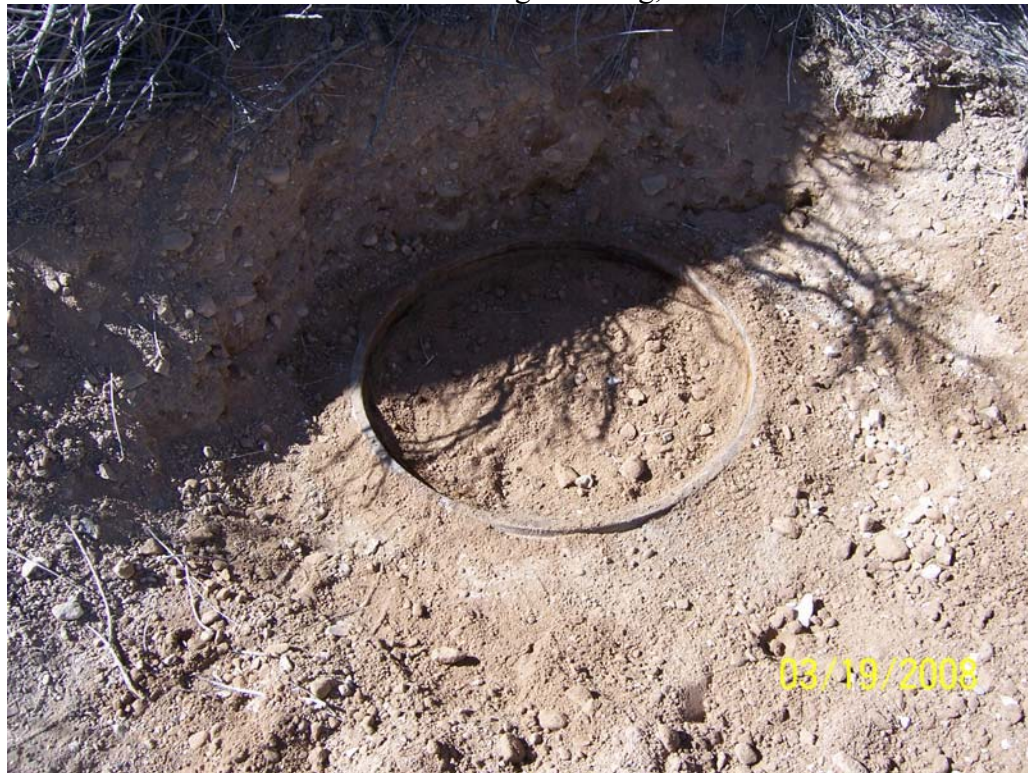
Photograph 28: CAS 12-04-01, System #4, Distribution Box after Grouting, 03/19/2008
