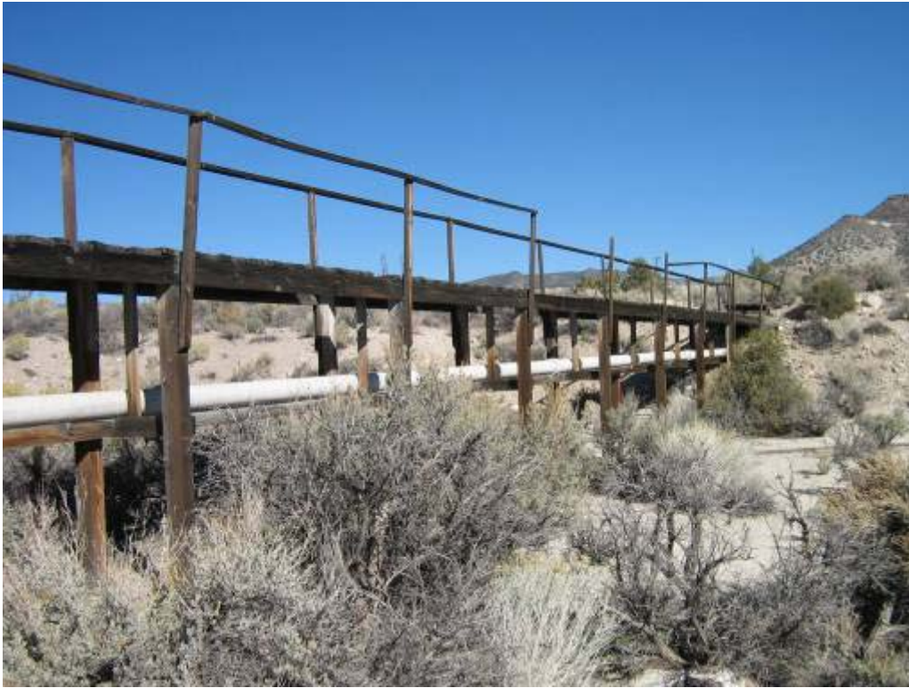
Photograph 1: CAS 18-03-01, Asbestos Cement Pipe and Wooden Walkway before Removal, 10/31/2007
