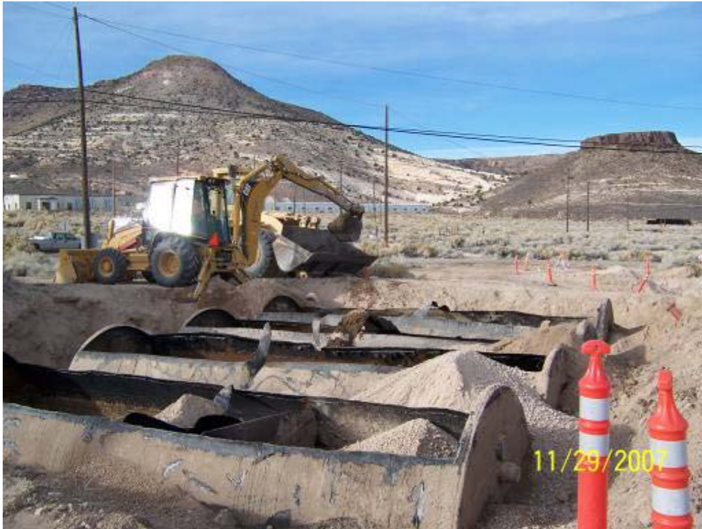
Photograph 14: CAS 12-04-01, Solidification of Sludge in System #4 Septic Tanks, 11/29/2007
