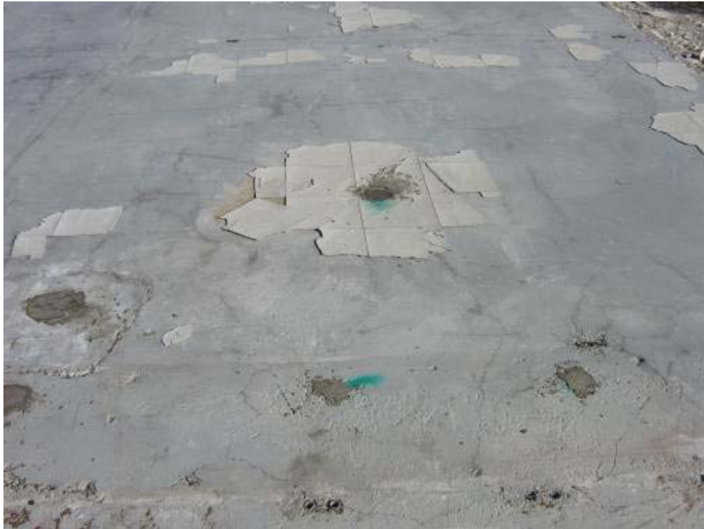
Photograph 12: Sewage Lines on Adjacent Concrete Pad in Area 12 Grouted, 11/28/2007
