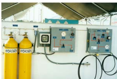
Small hydrogen refueling station for fuel cell neighborhood electric vehicles and fuel cell golf carts
