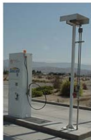
Hydrogen/Hythane® dispenser and leak protection system
