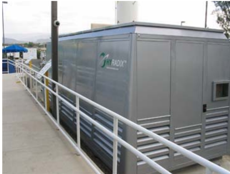
Figure 1 HyRadix Adéo™ Hydrogen Fuel Generator Installation at SunLine Transit Agency
