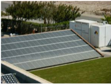
Solar panels provide energy to split water into the Stuart Energy Electrolyzer
