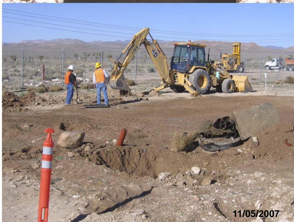
Figure D.1-9 Photographs of Inside Septic Tank and Removal of Orangeburg Leachpipe (CAS 11-59-01)
