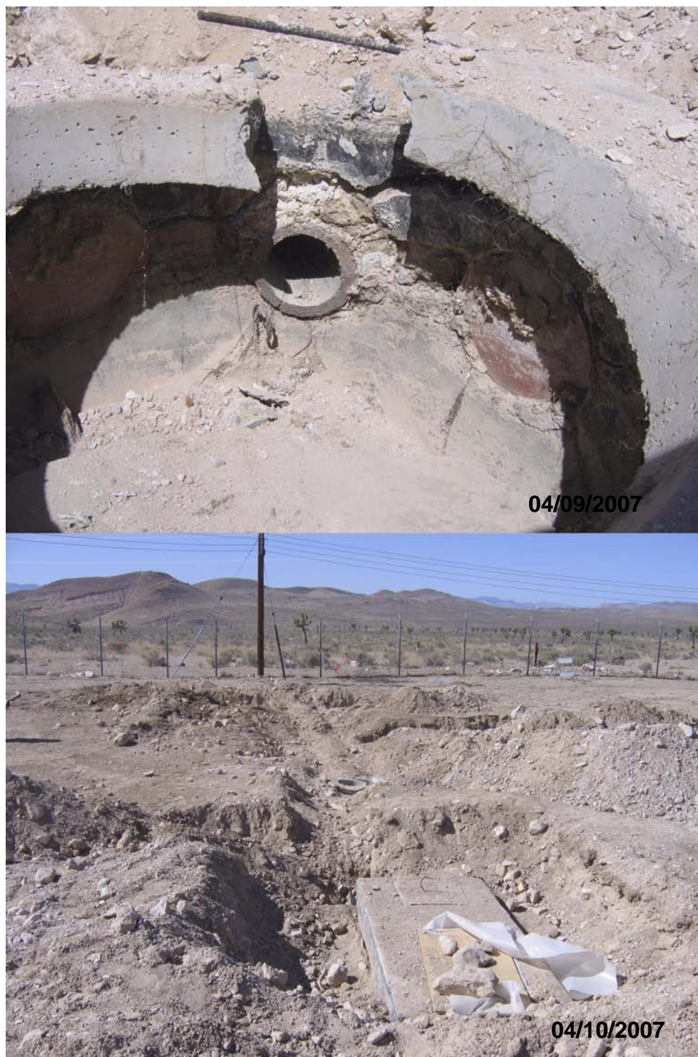
Figure D.1-8 Photographs of Uncovered Distribution Box and Septic Tank (CAS 11-59-01)
