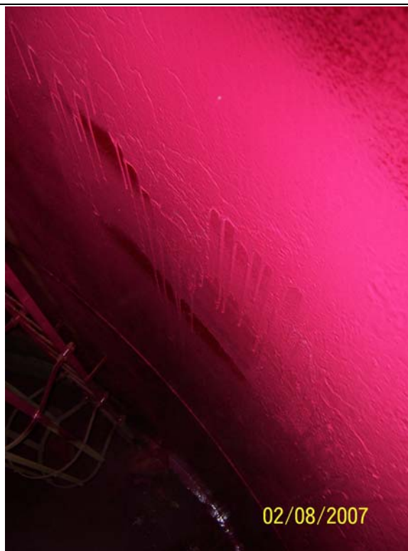
Photograph 3: CAS 25-01-05, Fixative on Interior of Aboveground Storage Tank, 02/08/2007
