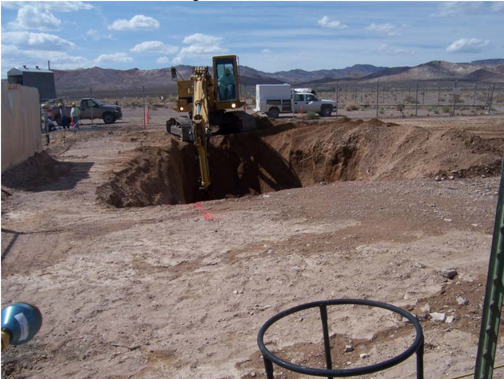
Photograph 14: CAS 25-02-02, Excavation of Overburden to Access Underground Storage Tanks, Facing Northwest, 05/21/2007
