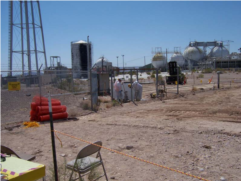
Photograph 24: CAS 25-23-11, Removal of Radiologically and Lead-Impacted Soil from Pump Vault, Facing West, 06/12/2007
