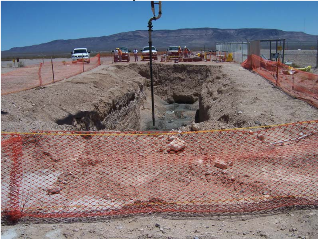
Photograph 16: CAS 25-02-02, Filling Underground Storage Tanks with Grout, Facing Southeast, 06/07/2007
