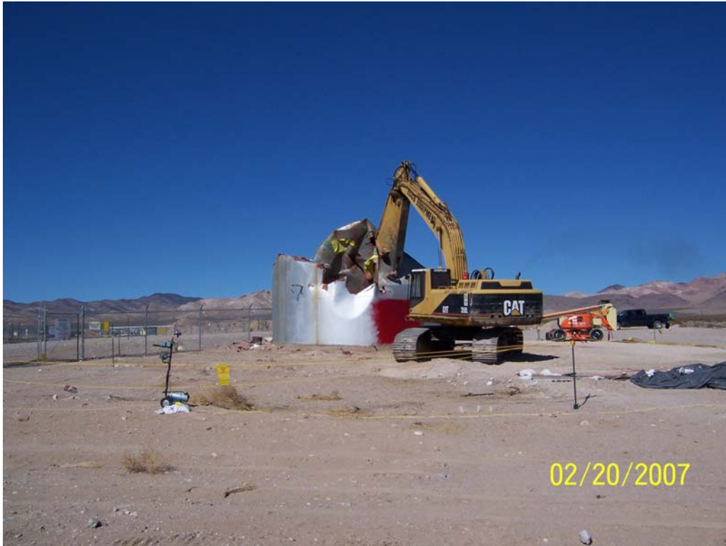
Photograph 5: CAS 25-01-05, Demolition of Aboveground Storage Tank, Facing North, 02/20/2007
