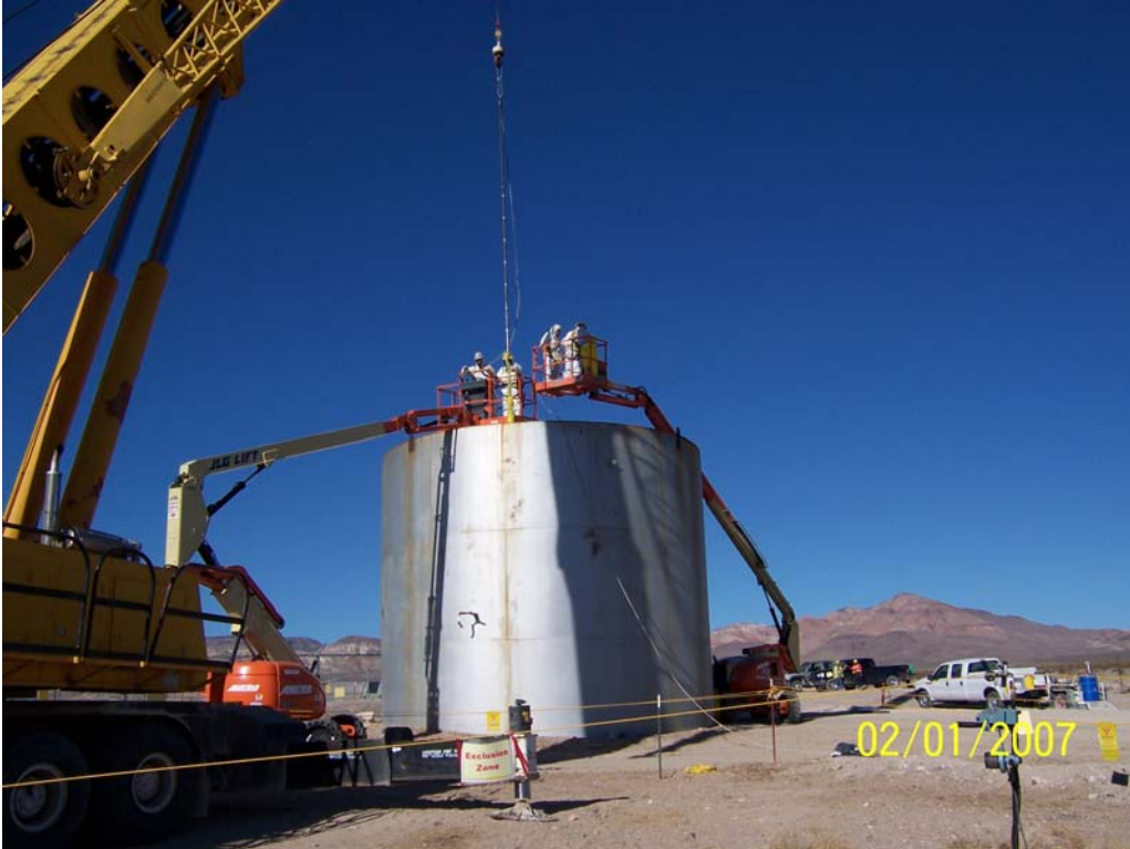
Photograph 2: CAS 25-01-05, Aboveground Storage Tank During Application of Fixative, Facing North, 02/01/2007
