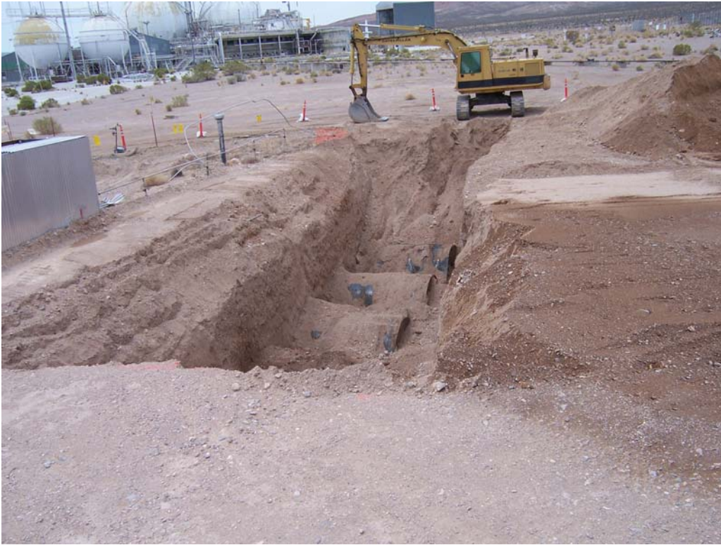
Photograph 15: CAS 25-02-02, Exposed Underground Storage Tanks, Facing West, 05/23/2007
