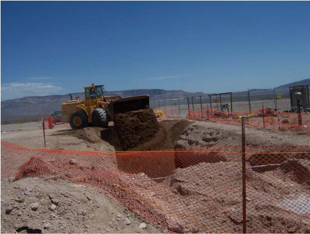
Photograph 17: CAS 25-02-02, Backfilling Underground Storage Tank Area, Facing Southeast, 06/11/2007
