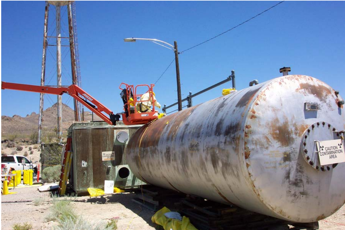
Photograph 29: CAS 26-01-01, Removal of Piping from Aboveground Storage Tank, Facing Northeast, 06/28/2007
