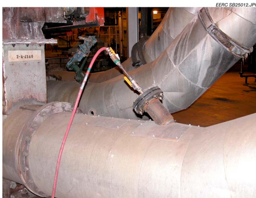
Figure 5-4. SEA injection lances shown installed at MRY Unit 2.
