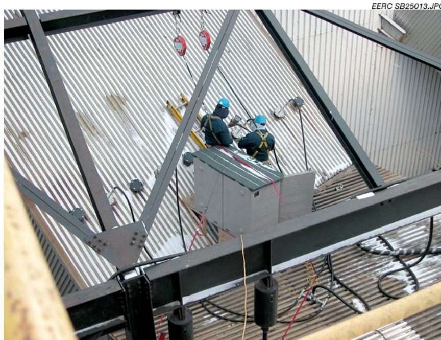
Figure 5-5. PAC injection and OH and CMM sampling locations.
