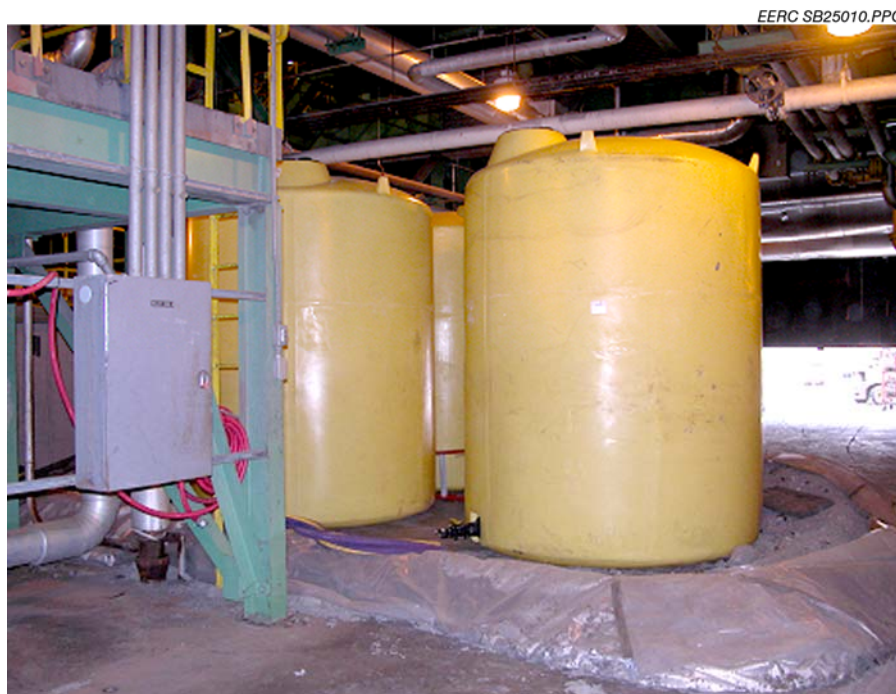
Figure 5-2. Oxidant or SEA storage tanks at MRY.
