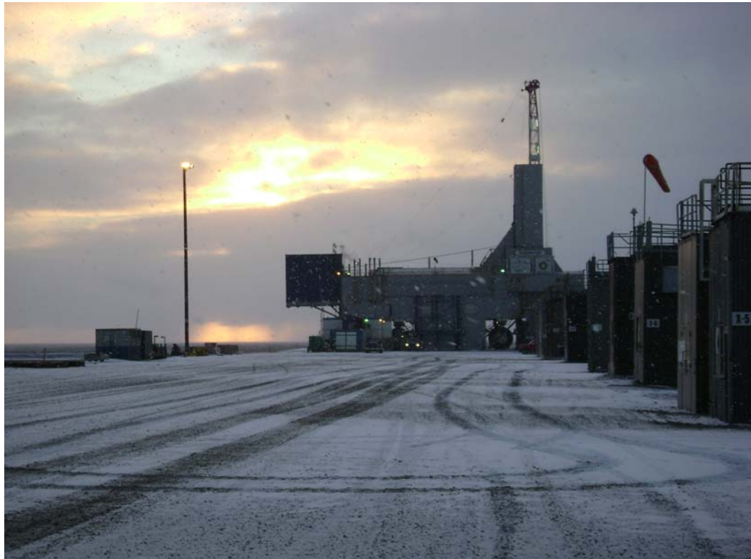
Photo 3: Nordic 2 Rig in Prudhoe Bay September 2007
