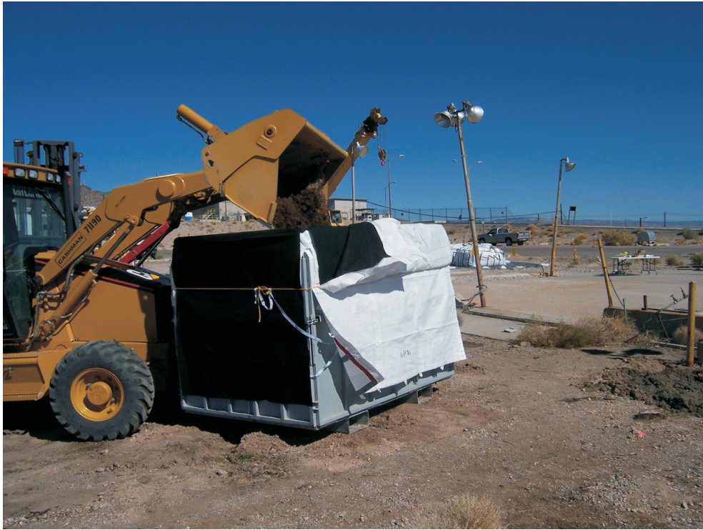
Photograph 19: Area 6 Decon System, Pu-soil during loading for disposal transport (07/20/2007)
