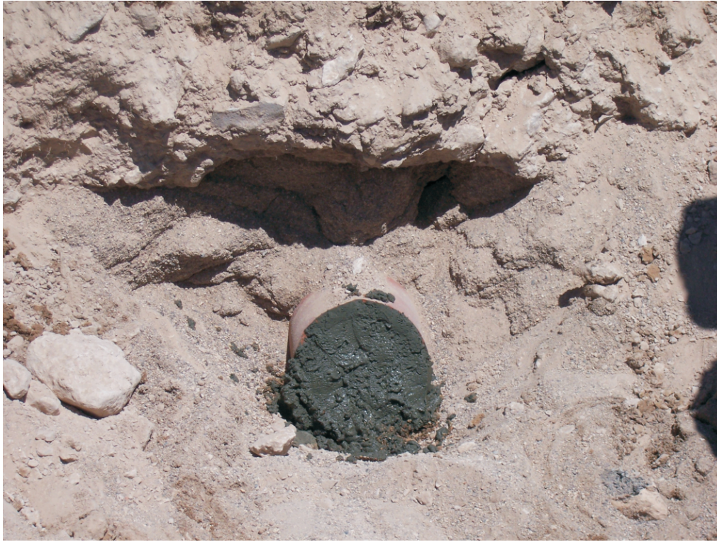
Photograph 25: CAS 11-04-01, Tank piping grouted in place (08/08/2007)
