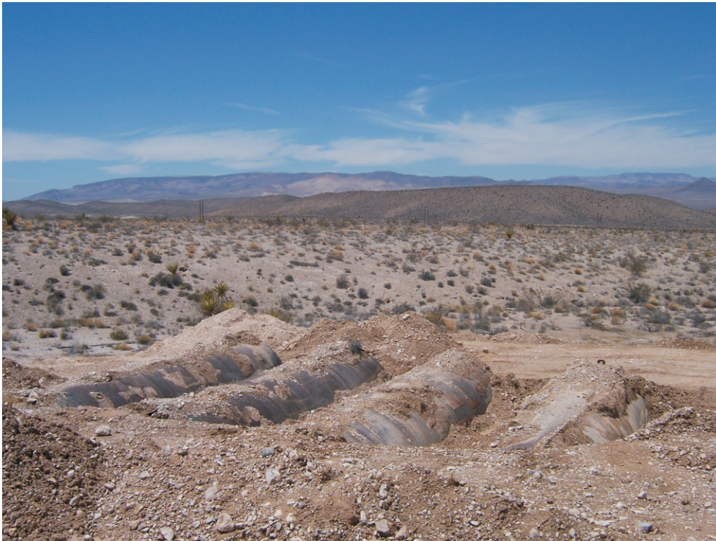
Photograph 5: CAS 05-04-01, Septic tanks exposed prior to removal (07/12/2007)
