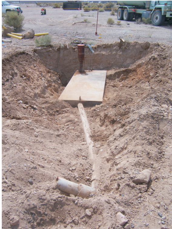
Photograph 1: CAS 02-04-01, Septic tank exposed during excavation (08/14/2007)
