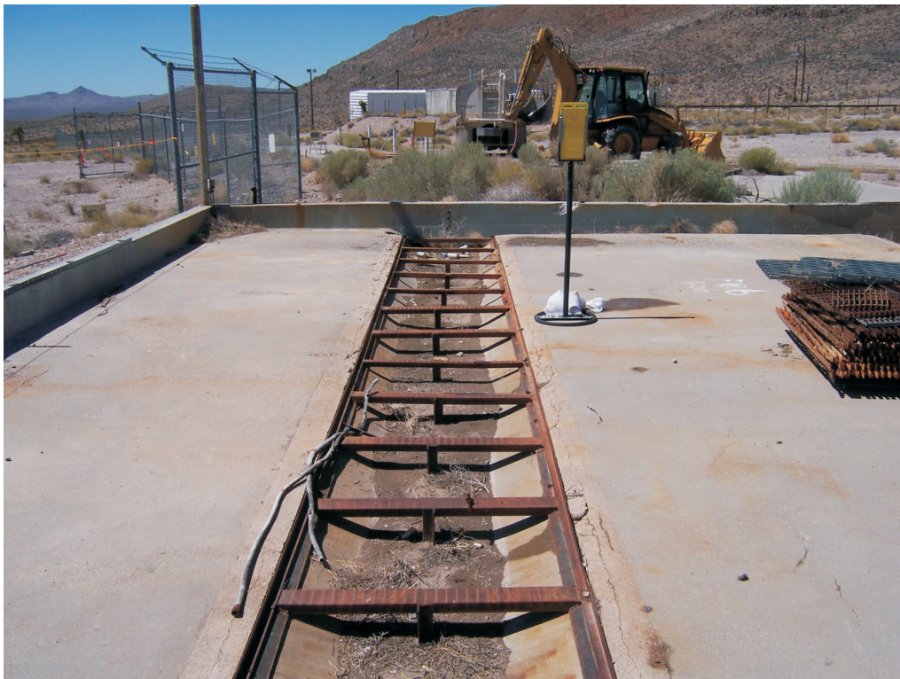
Photograph 10: Area 6 Decon System, Pad drain trenches with grating removed (07/19/2007)
