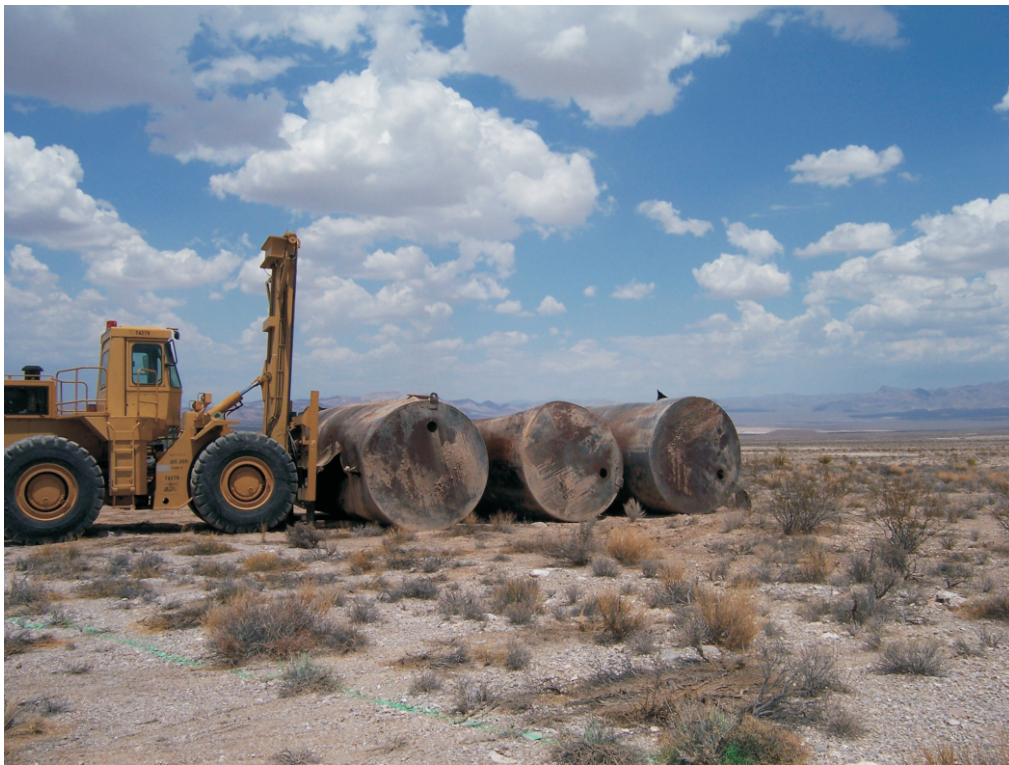
Photograph 6: CAS 05-04-01, Septic tanks during removal (07/25/2007)
