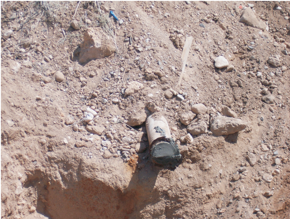
Photograph 2: CAS 02-04-01, Drain line pipe grouted after excavation (08/15/2007)
