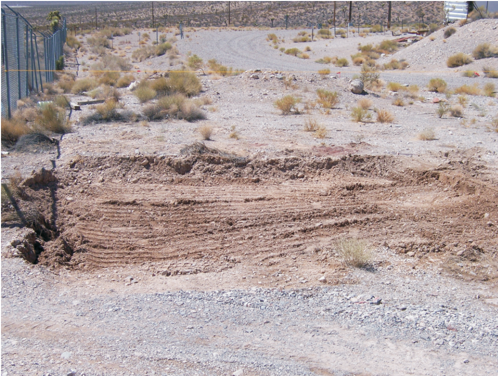
Photograph 18: Area 6 Decon System, Pu-impacted soil area during excavation (07/19/2007)
