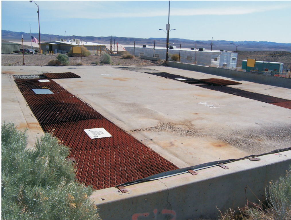
Photograph 9: Area 6 Decon System, Pad drain trenches prior to corrective action (04/19/2007)
