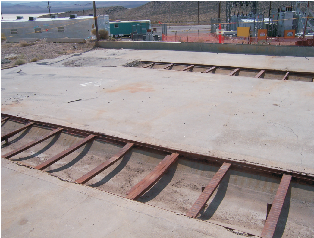
Photograph 12: Area 6 Decon System, Pad drain trenches after sediment removal (07/23/2007)
