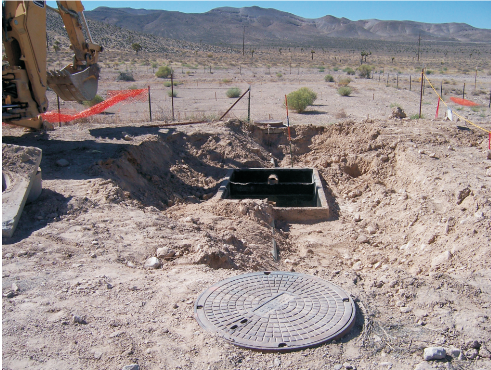
Photograph 23: CAS 11-04-01, Tank distribution box exposed (08/08/2007)
