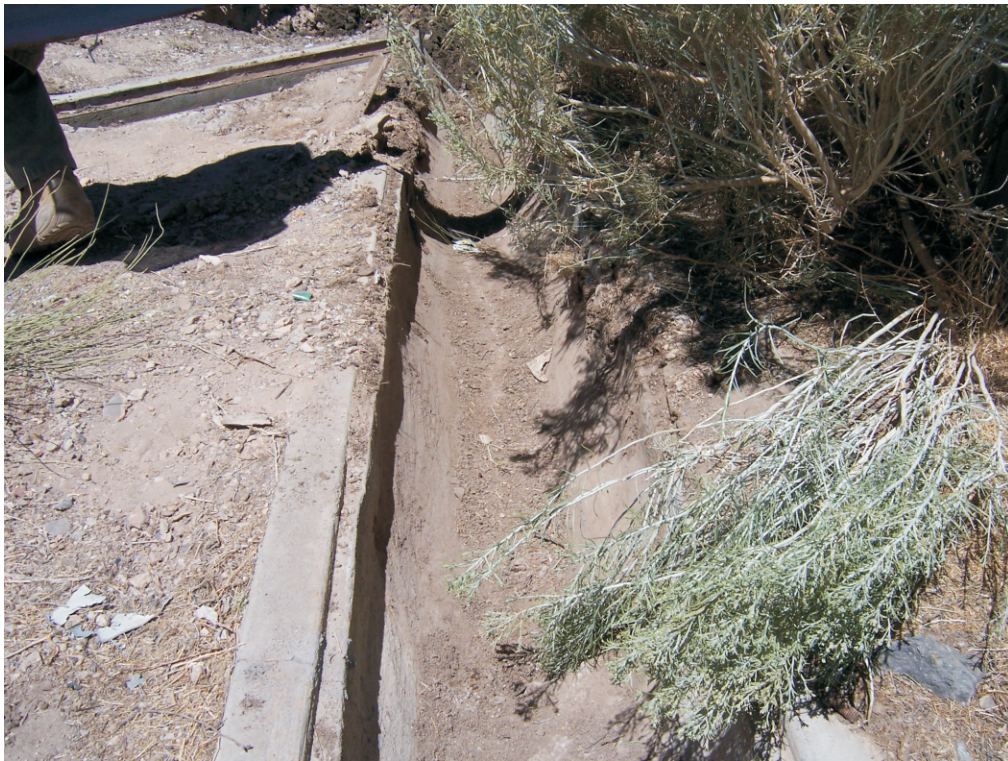
Photograph 15: Area 6 Decon System, Sump trenches after sediment removal (07/20/2007)
