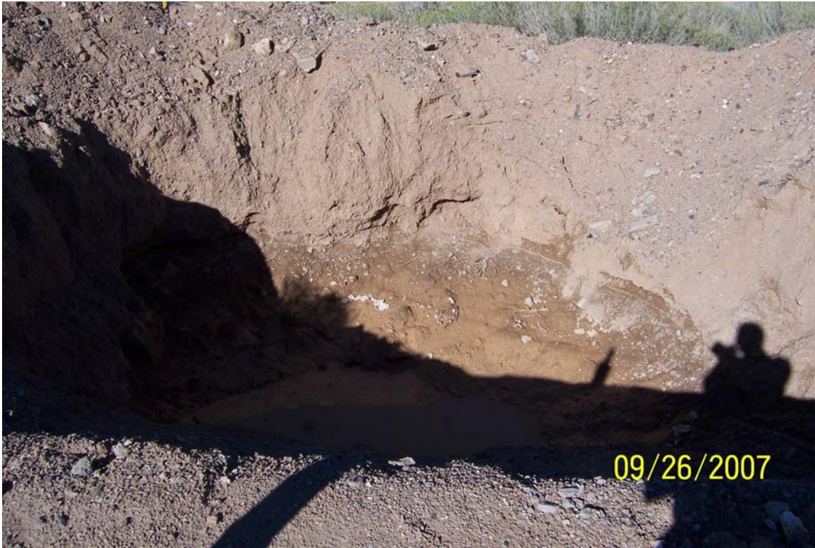
Photograph 5. CAS 06-07-01, Septic tank 6-607 excavation after tank removal
