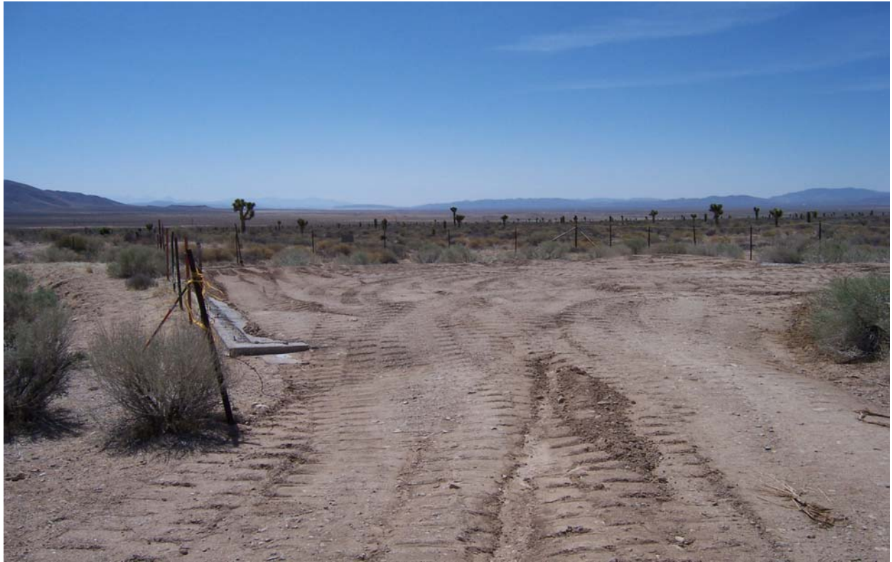
Photograph 49. CAS 15-23-03, Sump, partially filled, with concrete perimeter partially exposed
