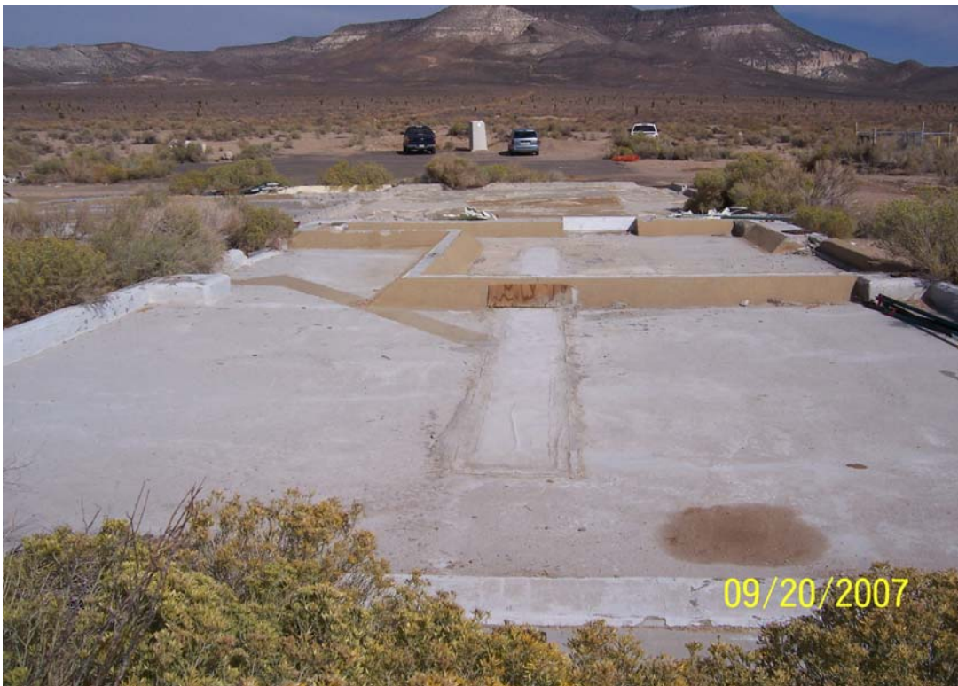
Photograph 34. CAS 15-01-03, Building 15-06 pad with floor drain trenches grouted
