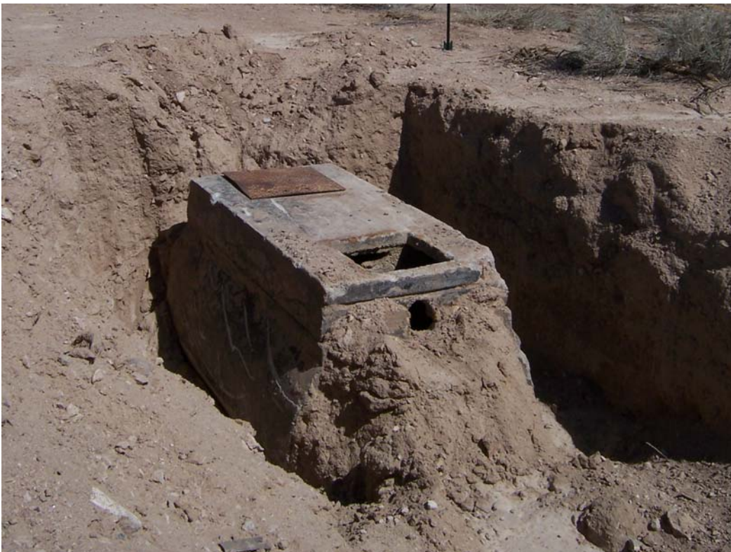
Photograph 42. CAS 15-04-01, Septic tank, excavated
