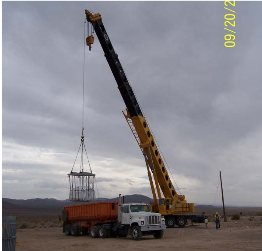
Photograph 31. CAS 15-01-03, Distribution box LLW loading onto transportation vehicle
