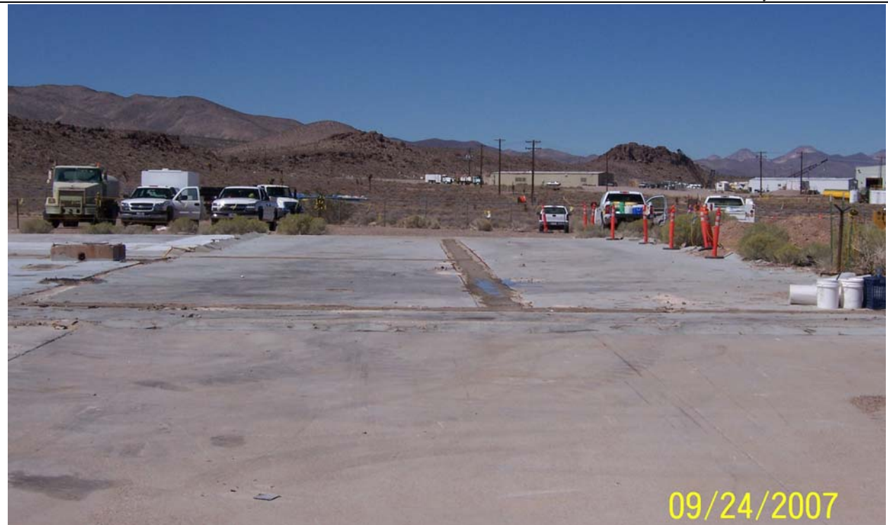
Photograph 13. CAS 06-07-01, Building 6-605 floor drain trenches, trenches grouted
