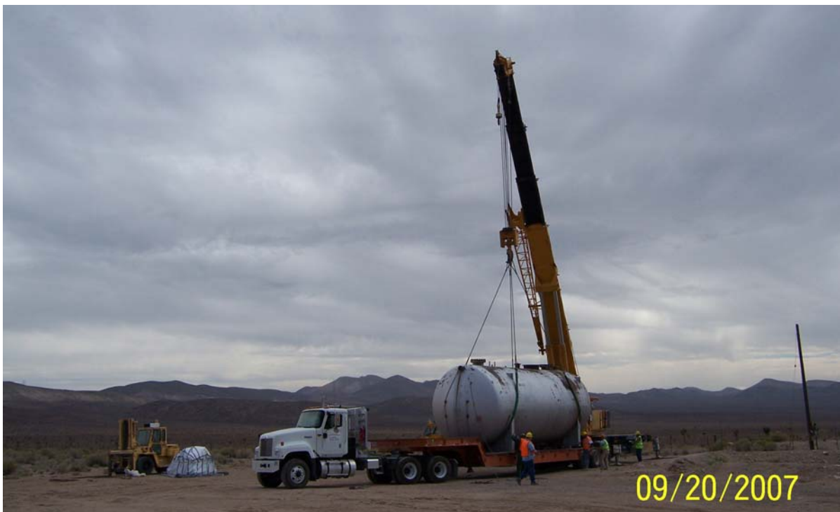
Photograph 24. CAS 15-01-03, Placing AST on flatbed trailer
