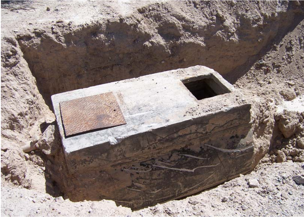
Photograph 41. CAS 15-04-01, Septic tank, exposed during closure activities
