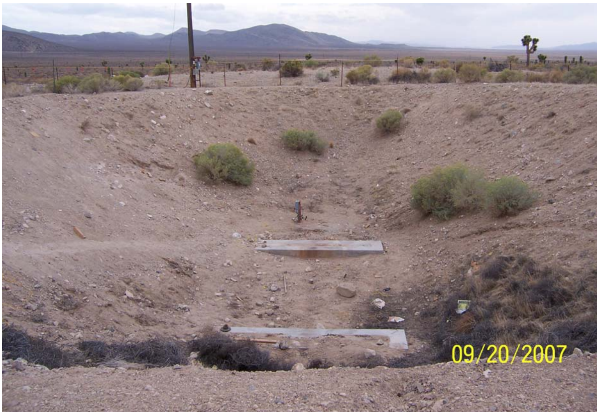
Photograph 26. CAS 15-01-03, AST depression after AST has been removed
