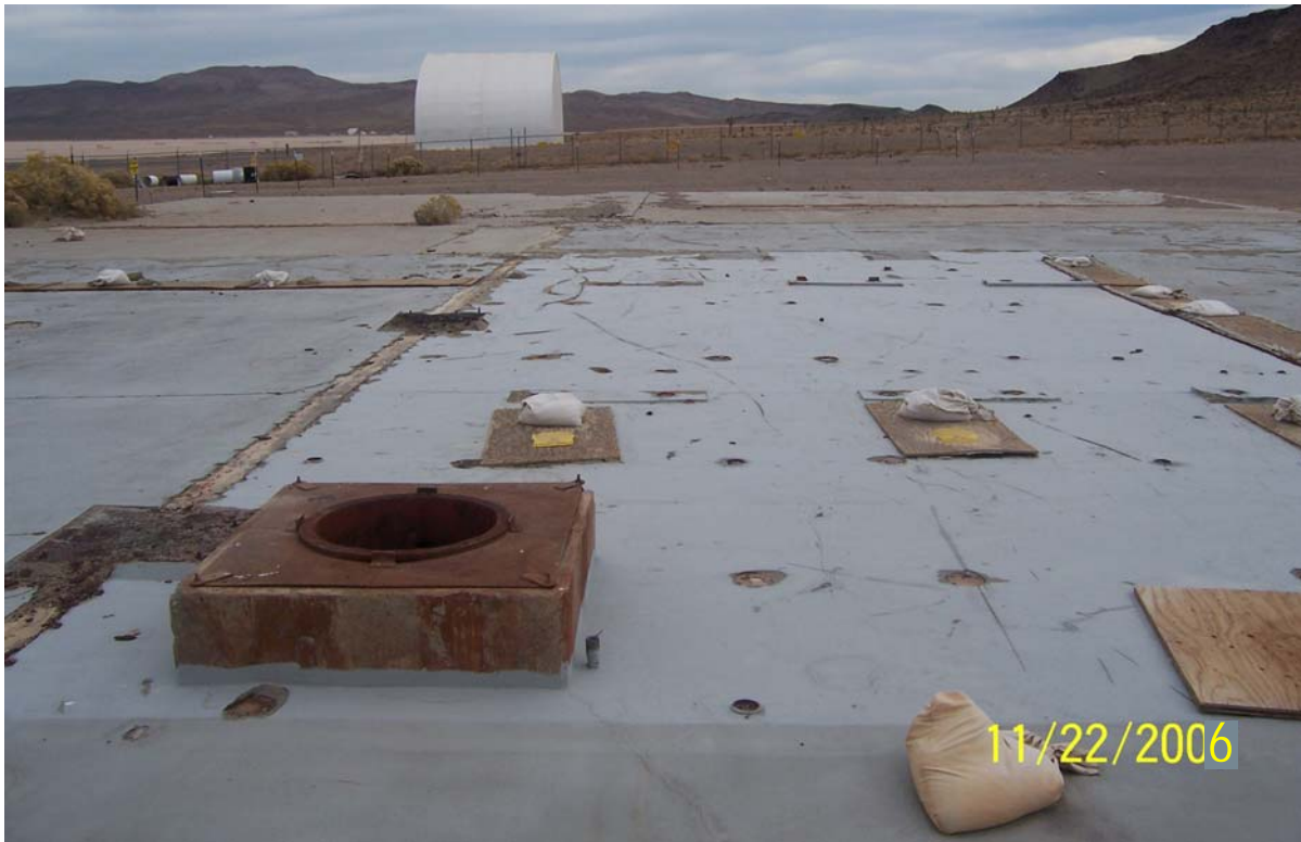
Photograph 11. CAS 06-07-01, Building 6-605 concrete pad, diversion box, trenches covered with plywood, before closure activities
