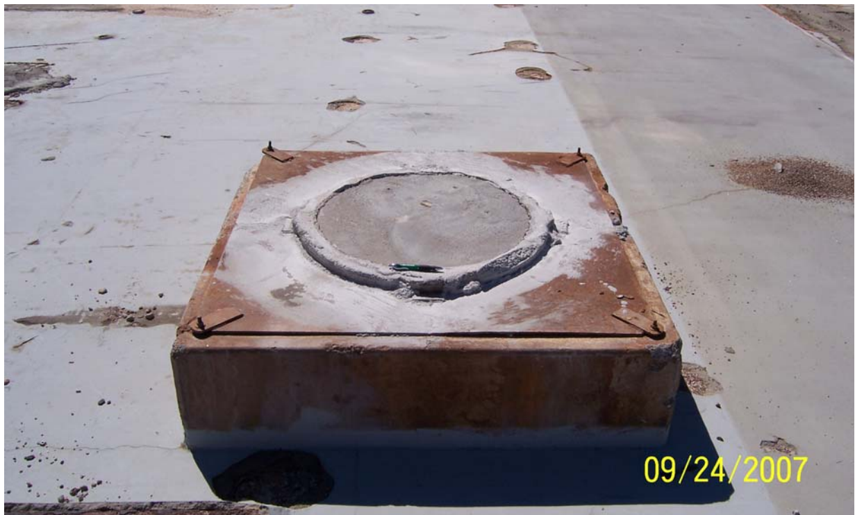
Photograph 12. CAS 06-07-01, Building 6-605 diversion box, grouted
