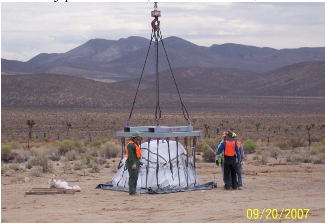
Photograph 30. CAS 15-01-03, Distribution box low-level waste (LLW) being prepared for lifting
