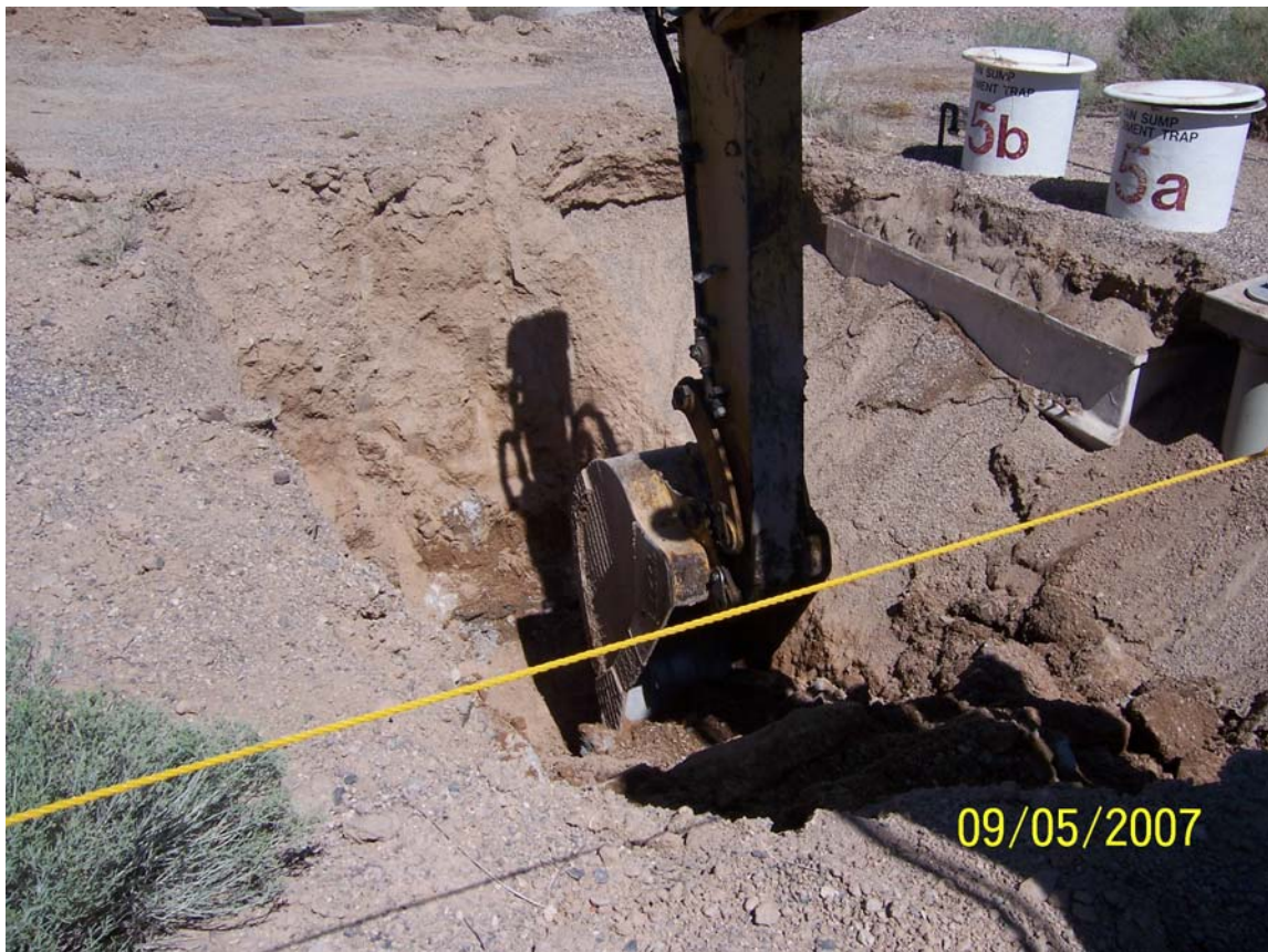
Photograph 7. CAS 06-07-01, Sump excavation, after sumps have been removed
