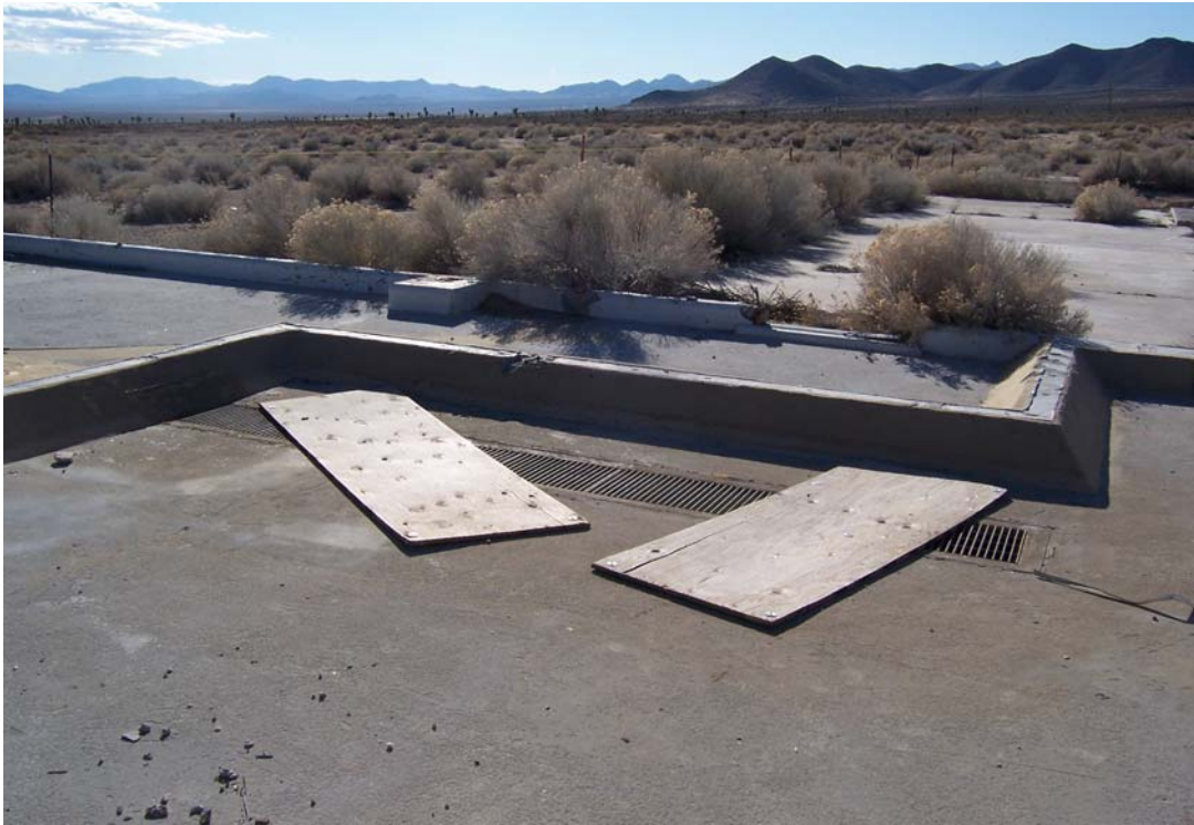
Photograph 33. CAS 15-01-03, Building 15-06 floor drain trenches, with wood debris, before closure activities
