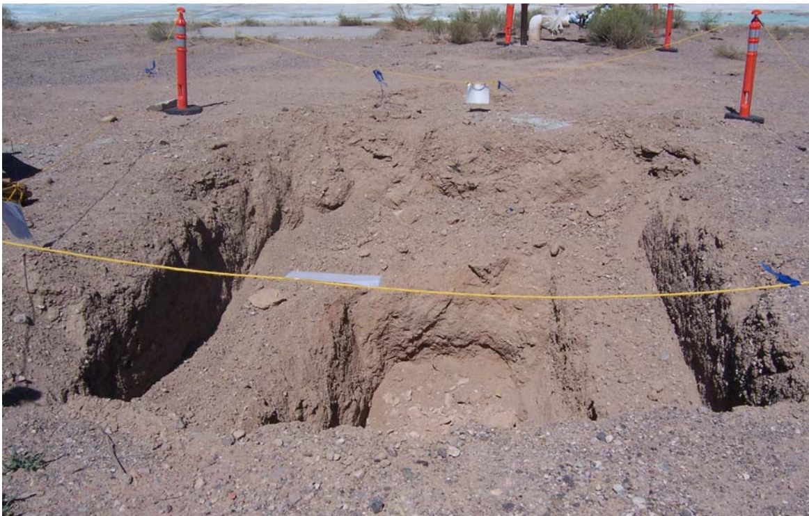
Photograph 2. CAS 06-07-01, Septic tank 6-605 excavation after tank removal
