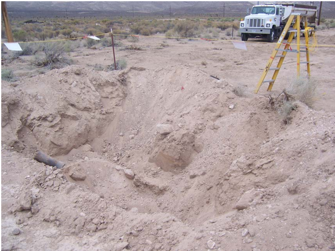
Photograph 28. CAS 15-01-03, Distribution box excavation, after box removal
