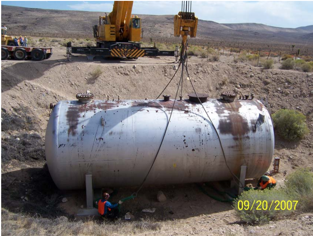
Photograph 23. CAS 15-01-03, Rigging AST for removal
