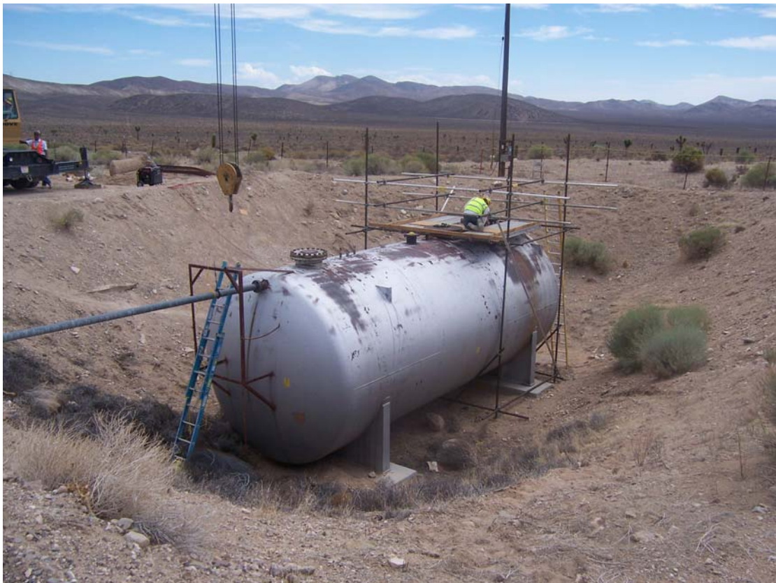
Photograph 22. CAS 15-01-03, AST scaffolding, checking tank contents
