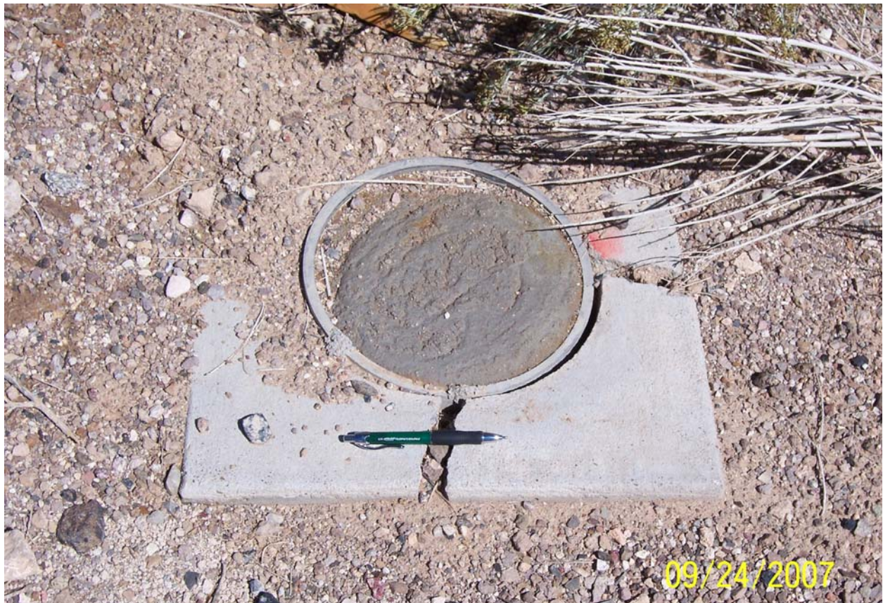
Photograph 10. CAS 06-07-01, Cleanout, grouted
