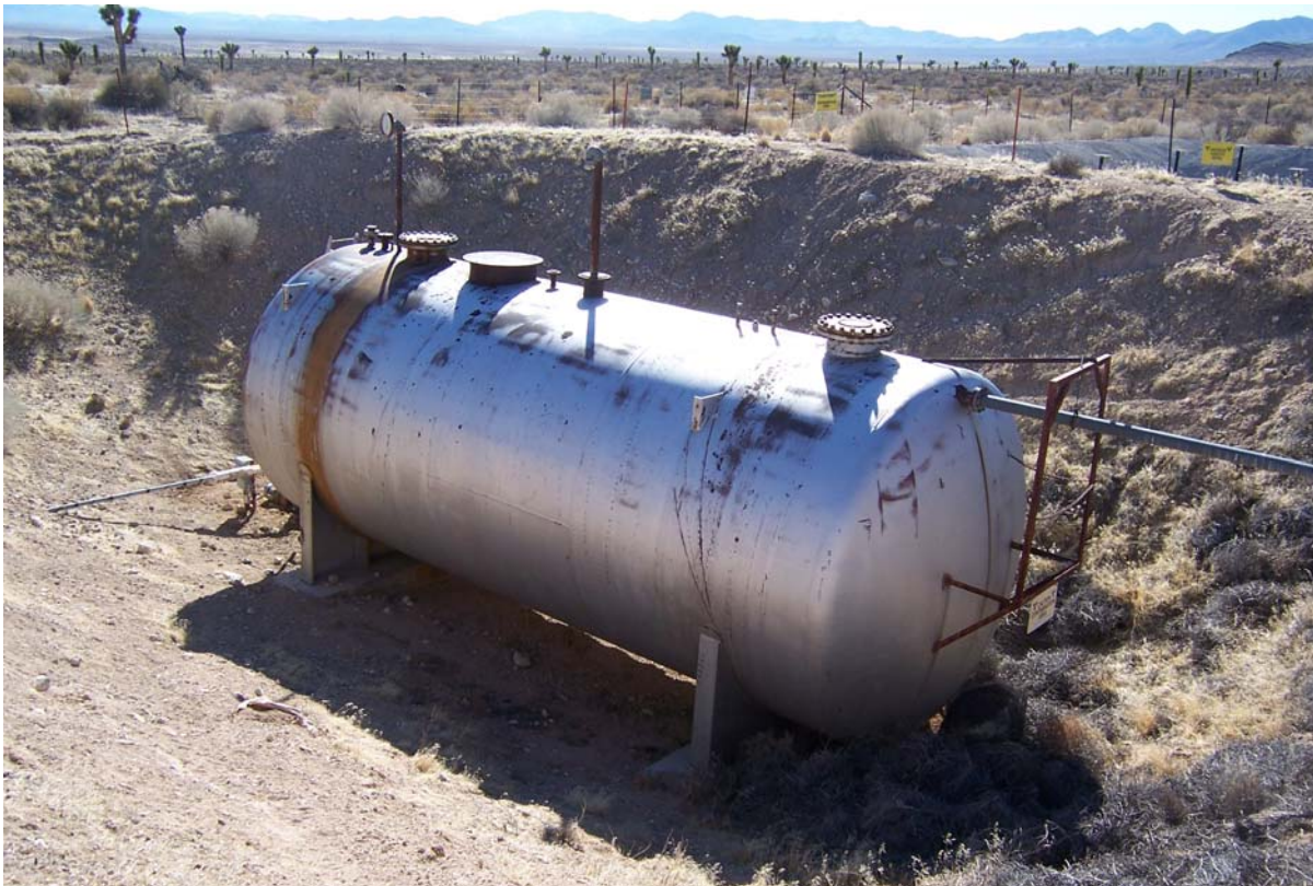
Photograph 20. CAS 15-01-03, Aboveground Storage Tank (AST), showing piping coming in from right (north) and going to fill stand (to east)
