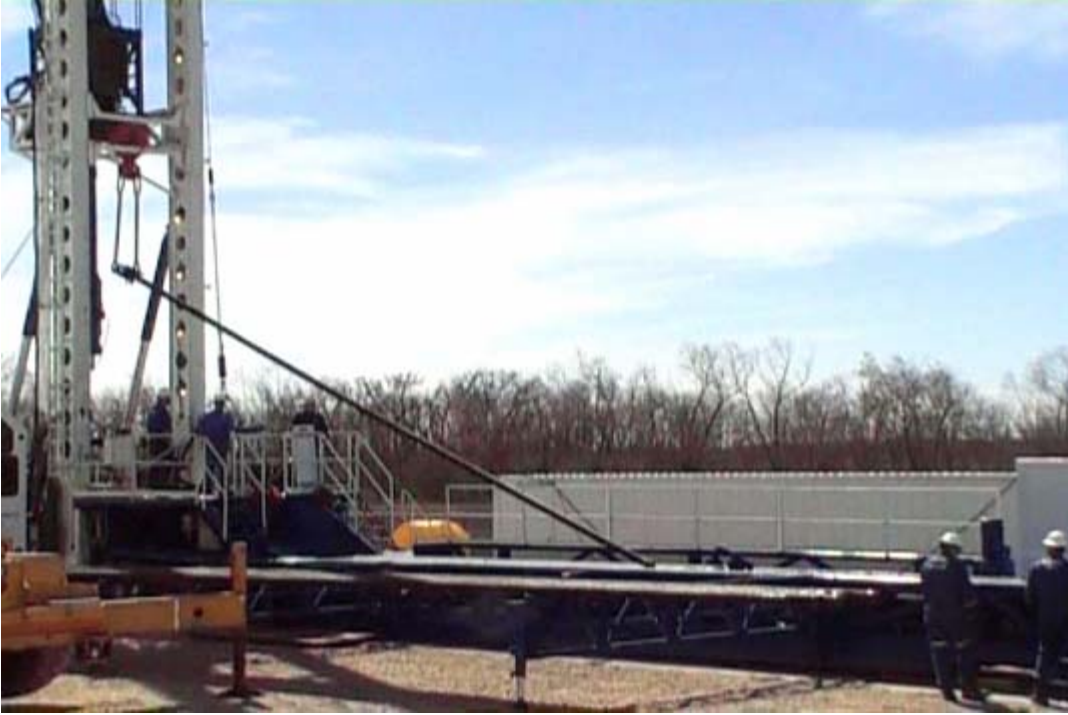
Figure 13-4 Laying down tubing
