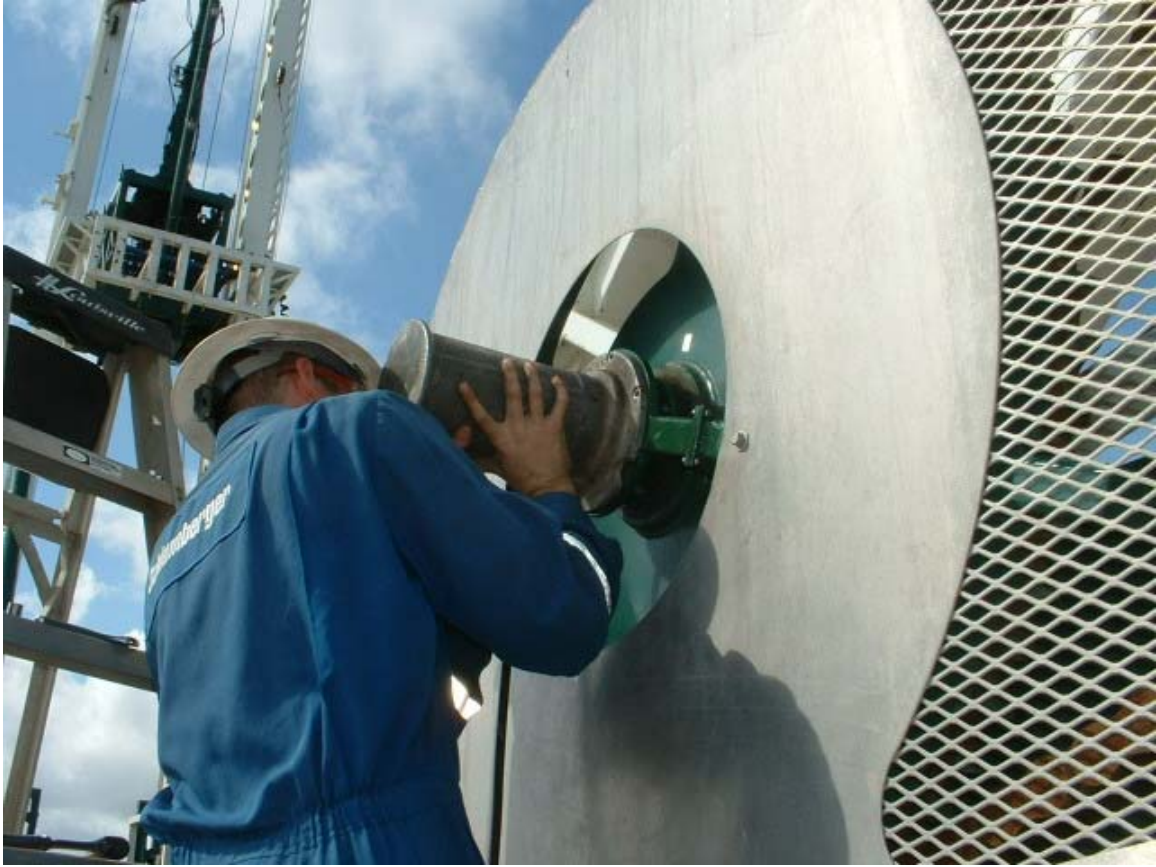
Figure 12-13 Showing installation of collector
