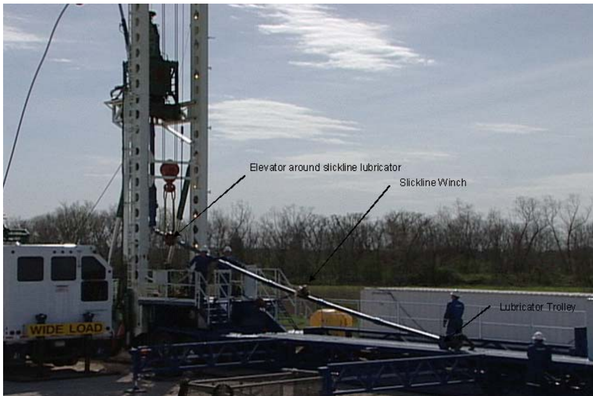
Figure 11-22 Raising slickline lubricator into derrick cont'd
