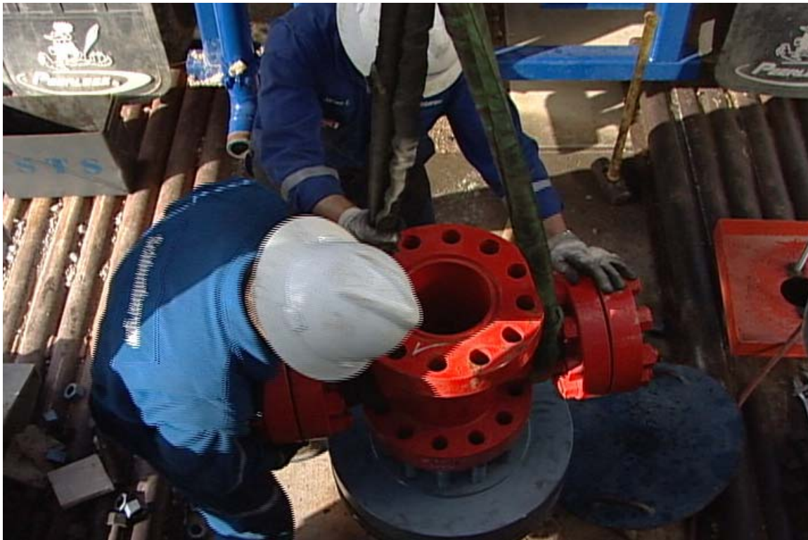
Figure 13-7 Flow cross being placed on well thru floor opening
