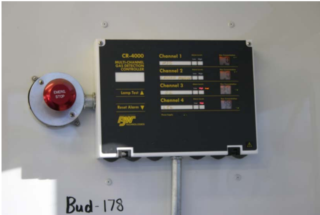
Figure 10-18 Gas detector display with emergency stop
