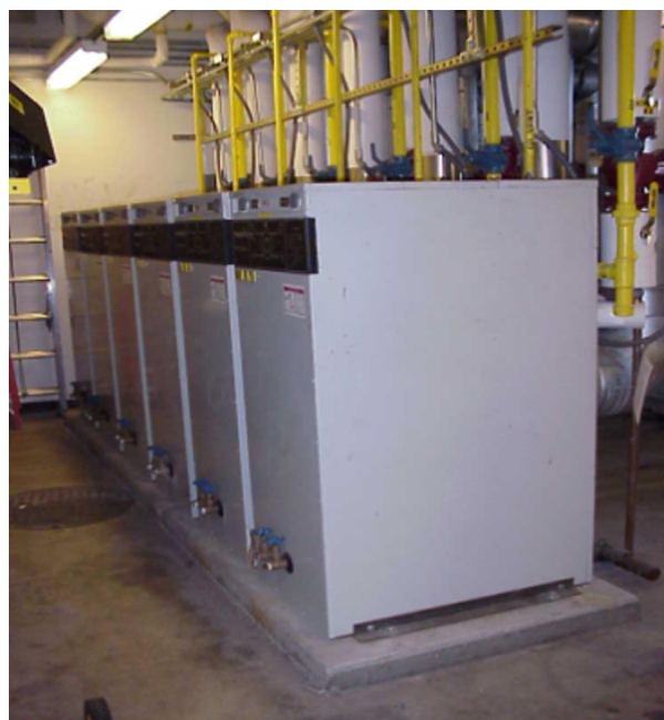
Figure 4. LBNL replaced two boilers with 11 modular boilers to maximize part-load efficiency.
