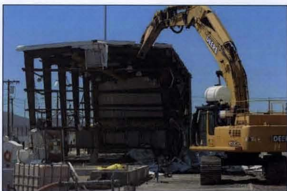
Excavator Pulling Down the 241-Z Structure
