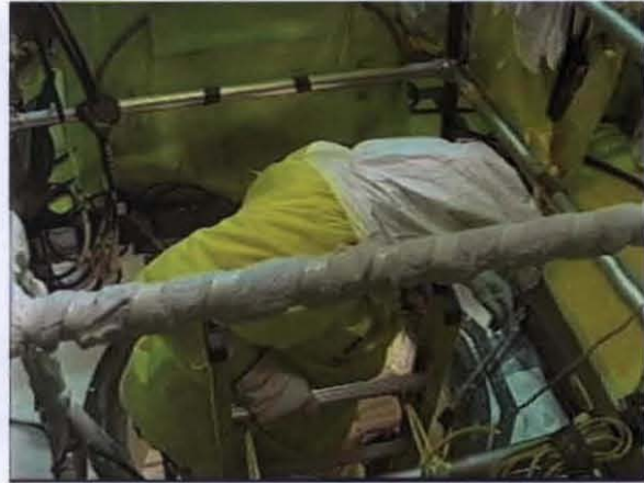
Worker Entering 241-Z Tank Vault Via 39" Opening
