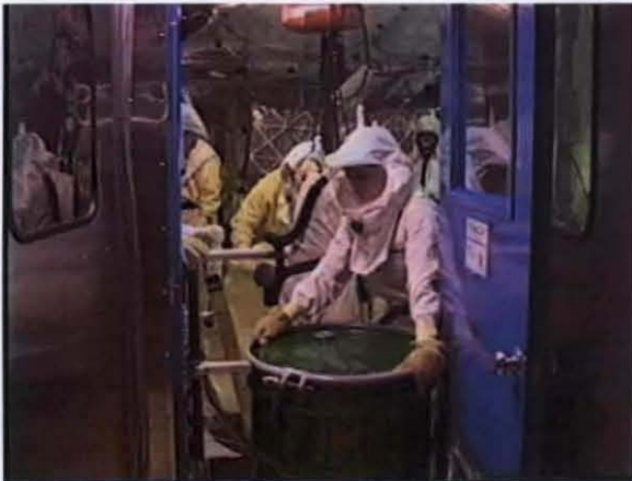
Removing Drum of Waste from Containment Tent
