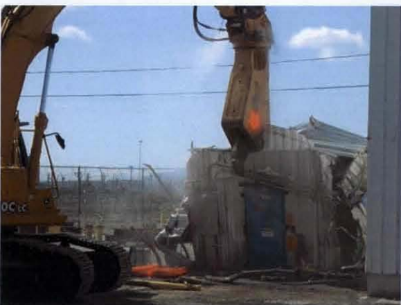
Demolition of 241-ZA Sample Building
