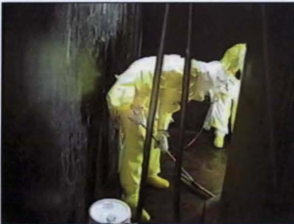
Cleaning a 241-Z Tank Vault Floor
