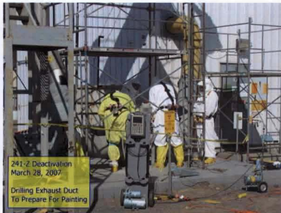
Preparing to Fix Contamination on Interior of 241-Z Exhaust Duct
