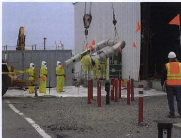
Removing 241-Z Exhaust Duct from Building to Load in to Special Transport Container
