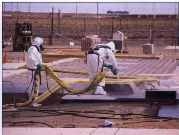
Installing Polyurea Environmental Barrier on 241-Z Slab
