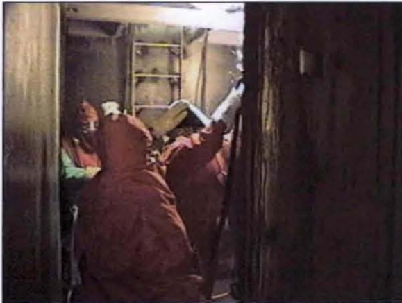
Using Plasma Arc Torch to Cut Access Opening in 241-Z Waste Tank
