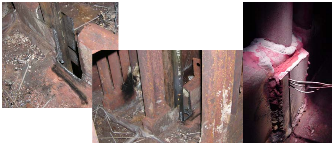
Figure 37. Photos showing the installation of superheater tube with strain gauges. In the picture on the left, the #2 tube has been installed in platen 14, but the hole is still empty where tube #1 with the strain gauges will be installed. In the center photo, the #1 tube with strain gauges is in position, and in the picture on the right, the tube is welded in place and the strain gauge and thermocouple wires extend through a specially made opening.
