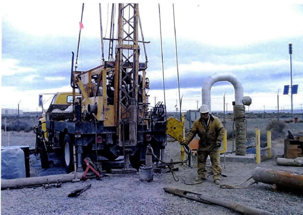
Fig. 2. A Fluor Hanford crew drills a well in the 200 Area of central Hanford, 2005.
