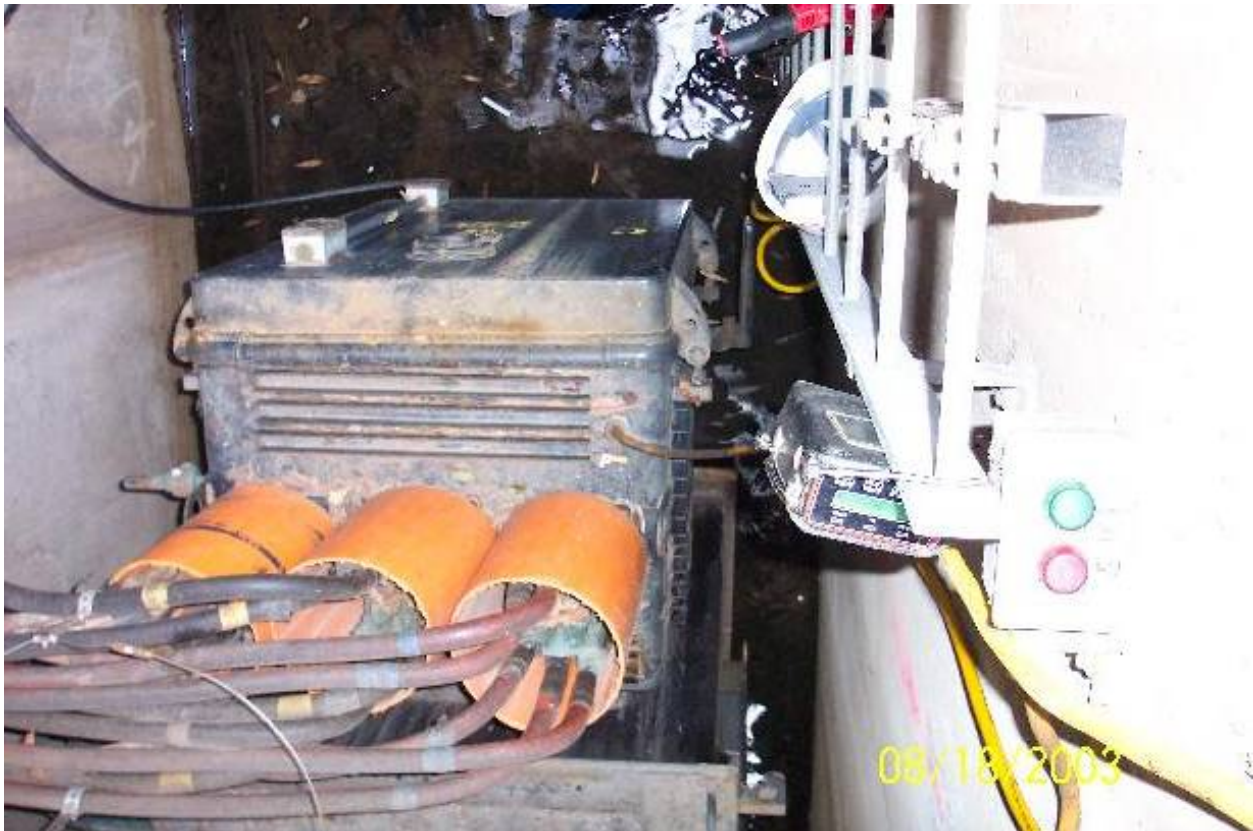
Figure 1: Network protector vault located below street level
