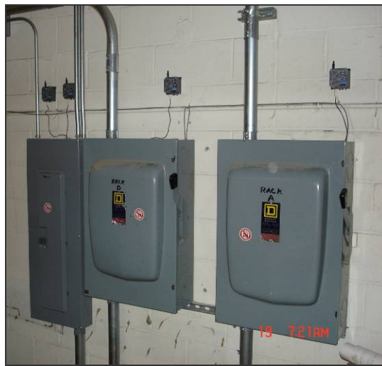
Figure 14. Motes connected to current transducers monitoring energy loads in building sub panels.
