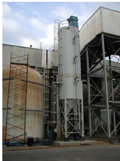
Figure 2-5. Carbon Injection Storage Silo/Feeder Train (Long-Term Testing)
