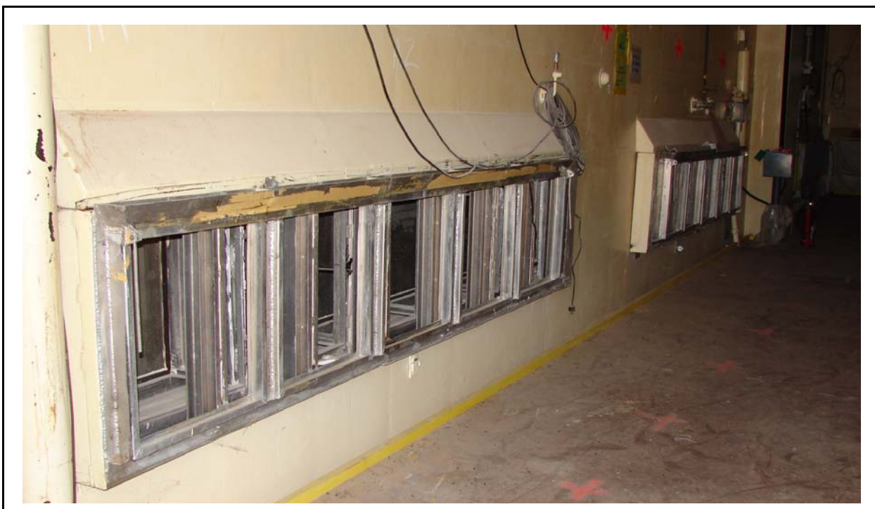
Figure 4-2 Filter Plenum in Room 107 (July 2007)
