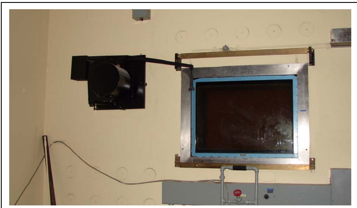
Figure 4-1 Observation Window (Leaded Glass) in Room 105 (July 2007)
