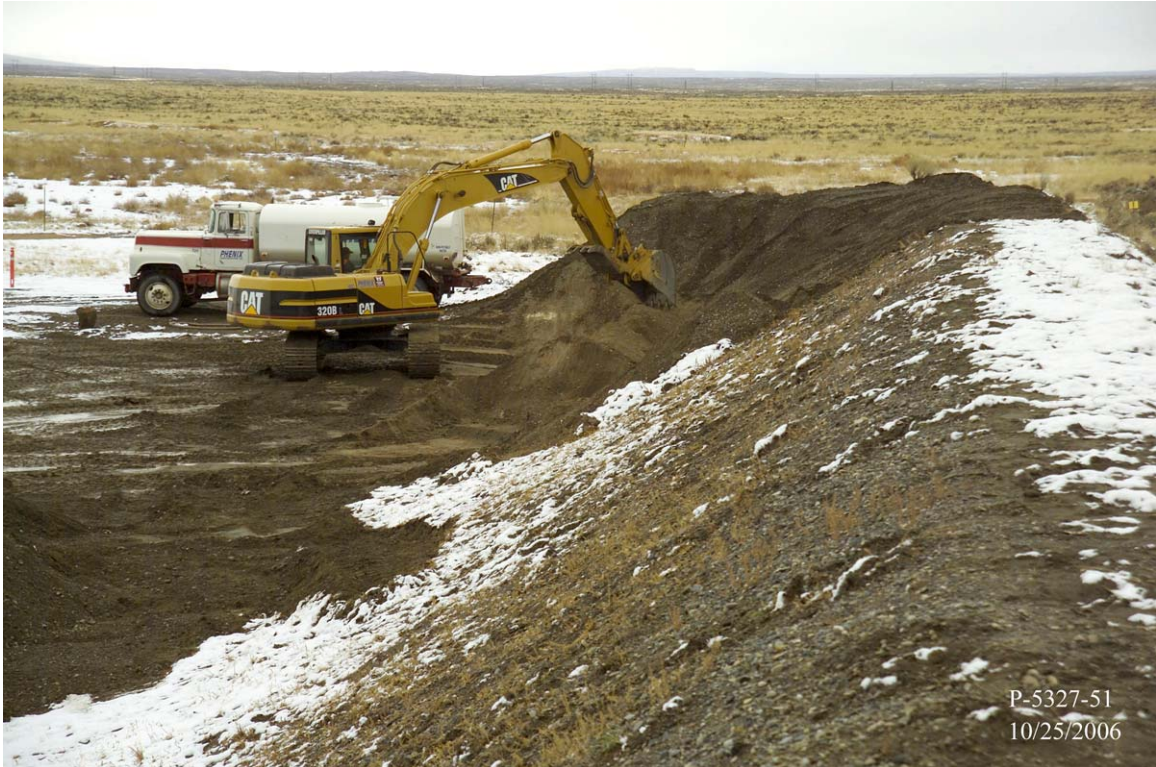
Figure A-19. Excavation of Berm B prior to screening.
