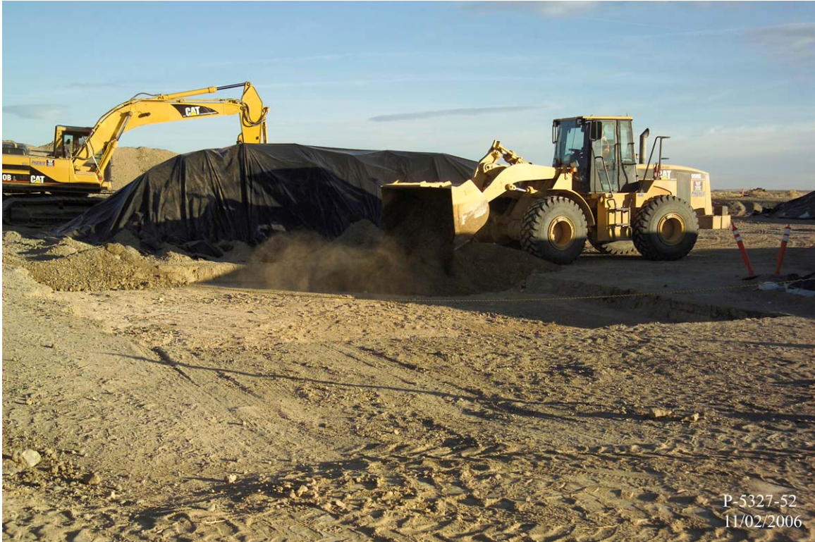
Figure A-20. Excavation of contaminated location between the berms.
