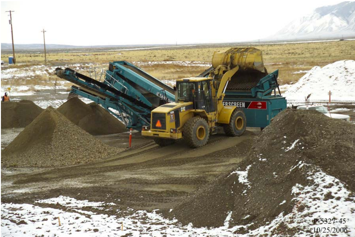
Figure A-18. Loading contaminated soil into the screening plant.
