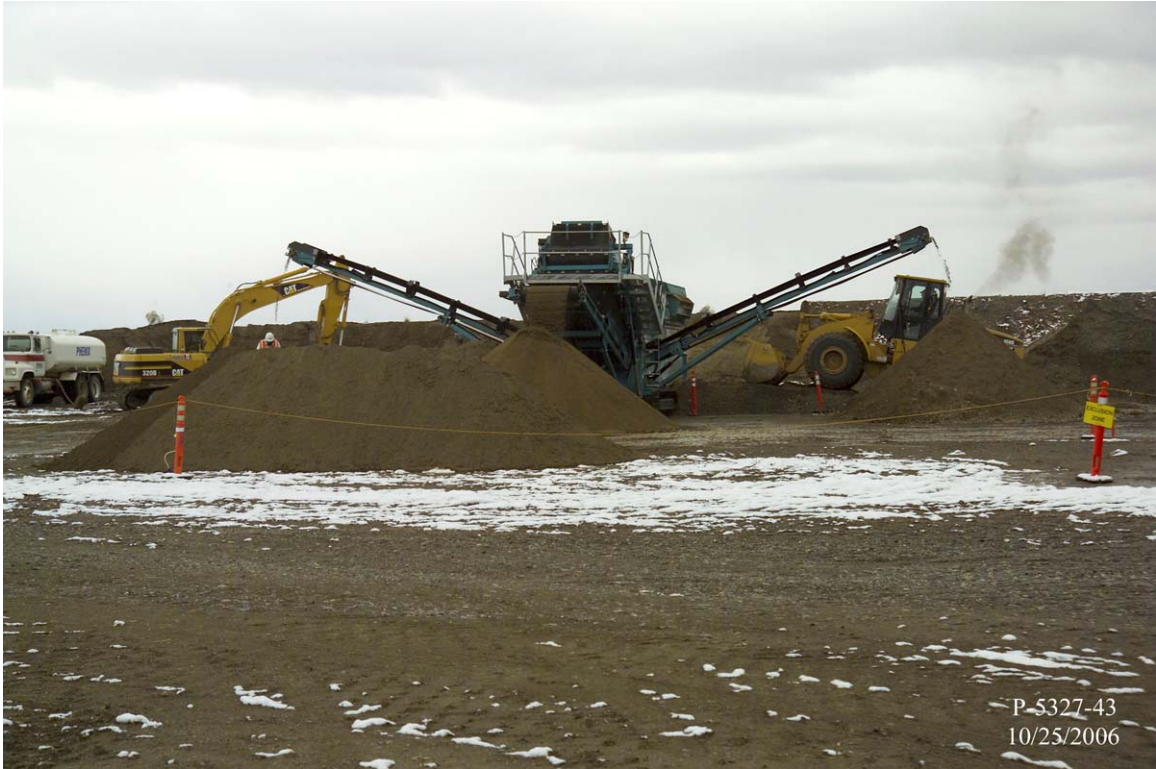
Figure A-16. Screening of lead-contaminated soils.
