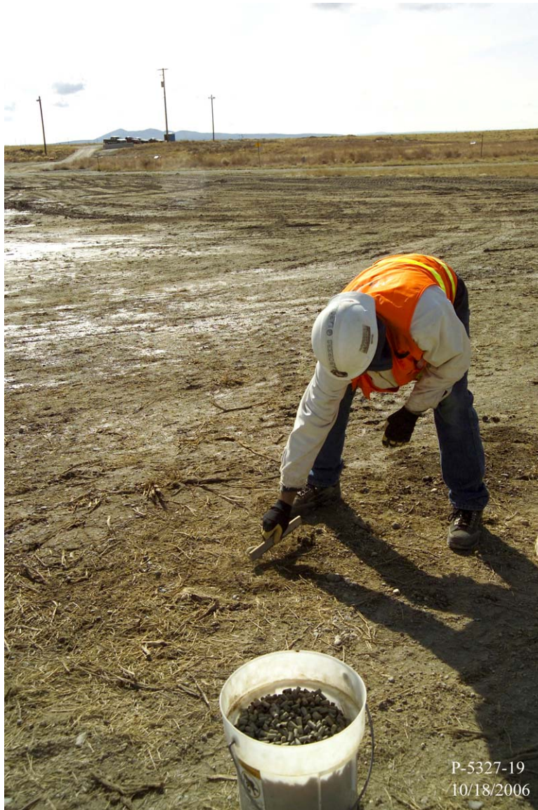
Figure A-9. Removing spent ammunition casings by hand.
