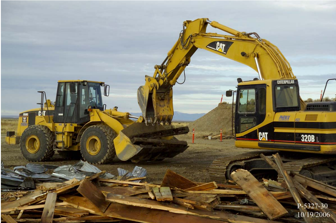
Figure A-12. Segregation of lead-contaminated railroad ties.
