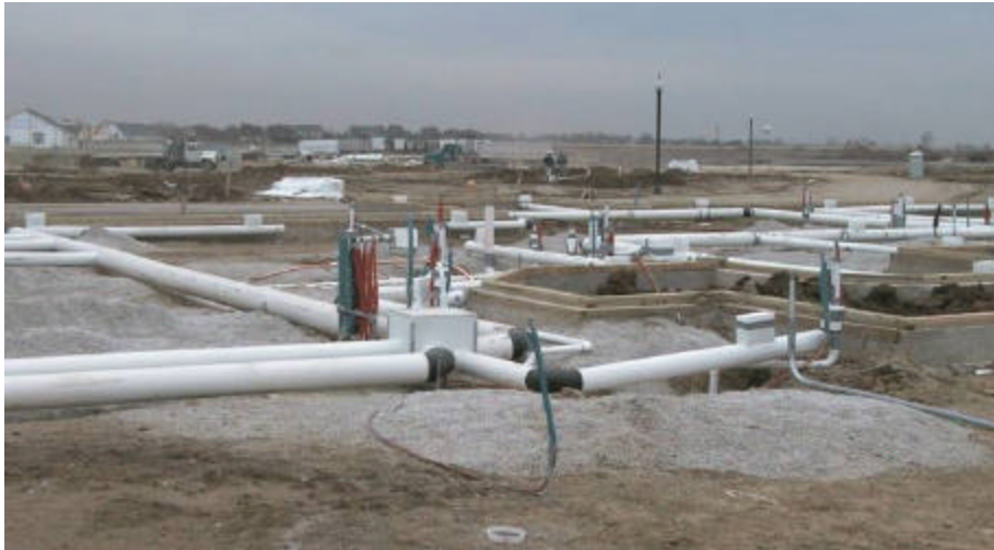
Plastic (PVC) ducts in the Chicago area prior to pouring of slab foundation.
