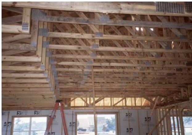
Figure 1 Recessed-configuration trusses in house designed by SWA for Mercedes Homes. The recesses allow for ductwork to be installed under the insulation layer, i.e., within the building's thermal envelope.
