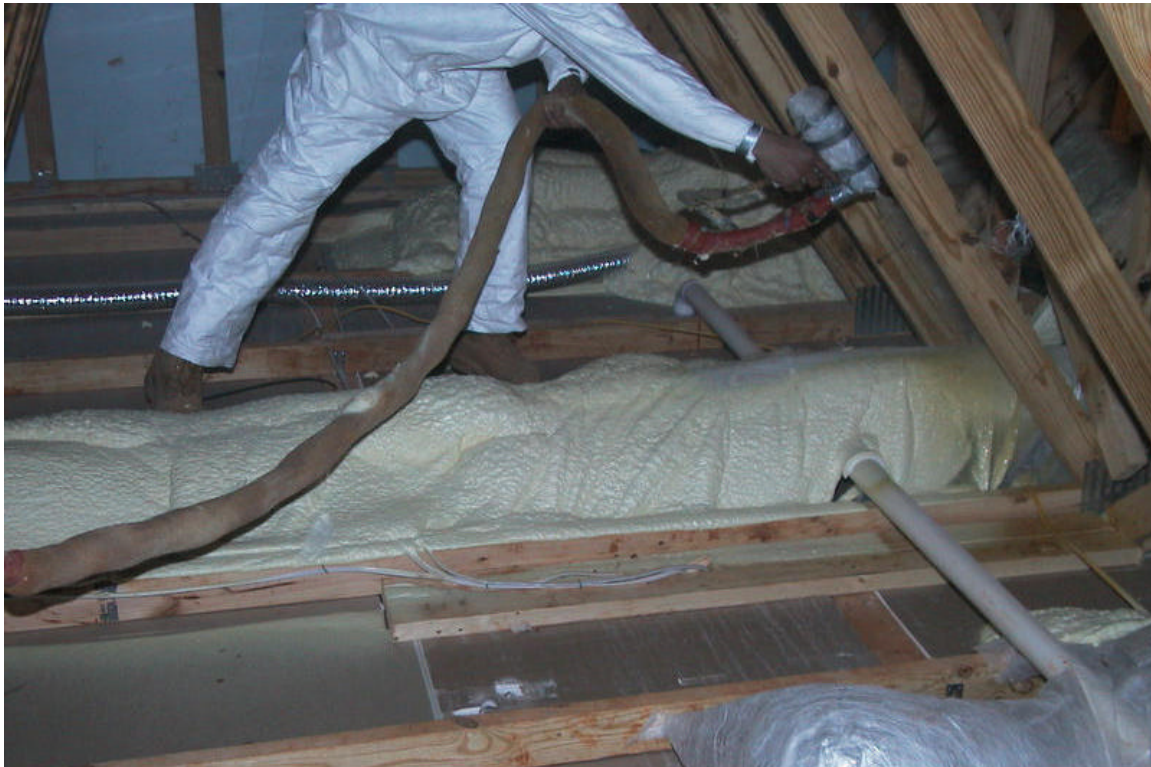
Application of polyurethane foam prior to blowing attic insulation in another Outlook home.
