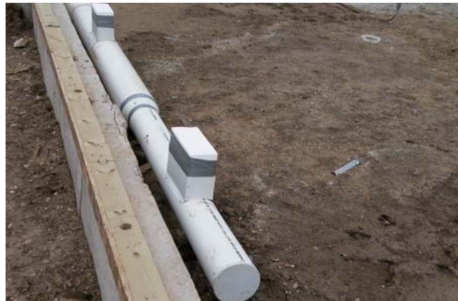
Figure 19 Underground PVC ductwork showing mechanical fastening of boot, often a source of leaks. Note the procedure for duct diameter reductions: transfer sections with taped joints, also subject to leaks.
