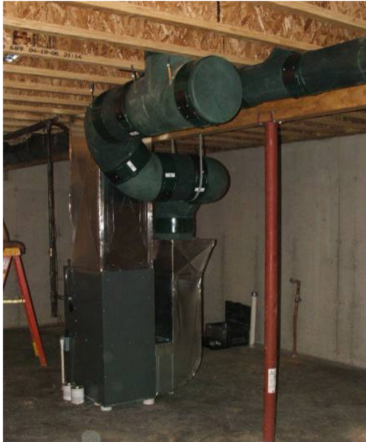
Supply Trunk and Return Plenum
