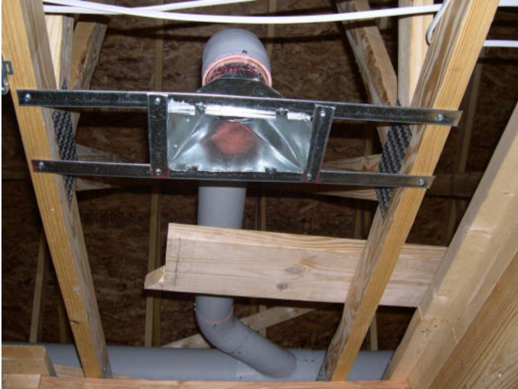
Branch take-off to register boot.
