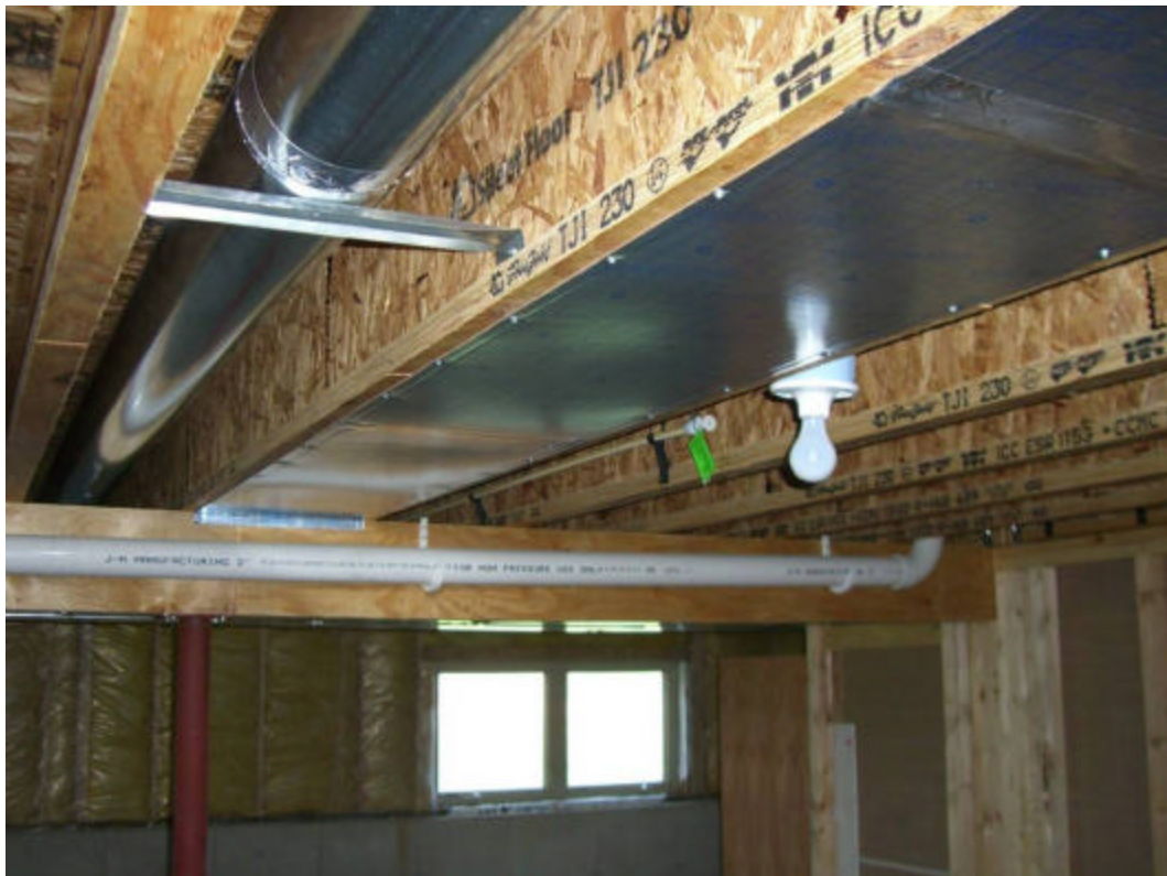
Sheet metal system with panned return in control house.
