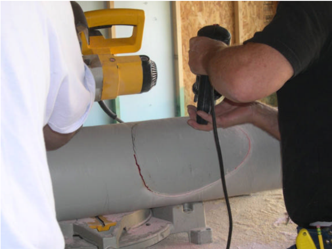
Cutting opening for saddle-type take-off.
