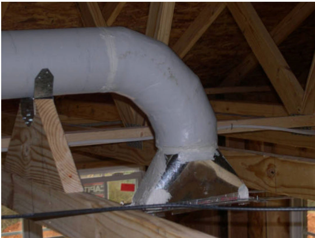
Duct support and turn to conventional register boot.
