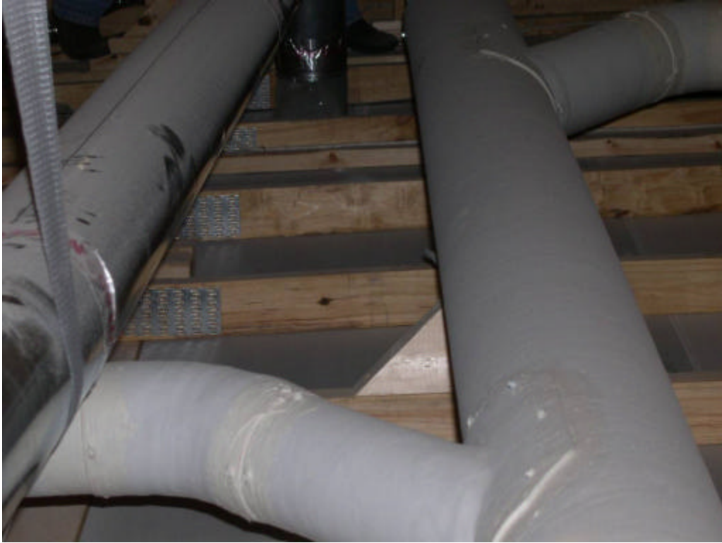
Joints covered with fiberglass tape and mastic.
