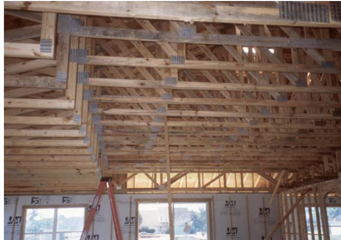
Figure 9 Recessed-configuration trusses in house designed by SWA for Mercedes Homes
