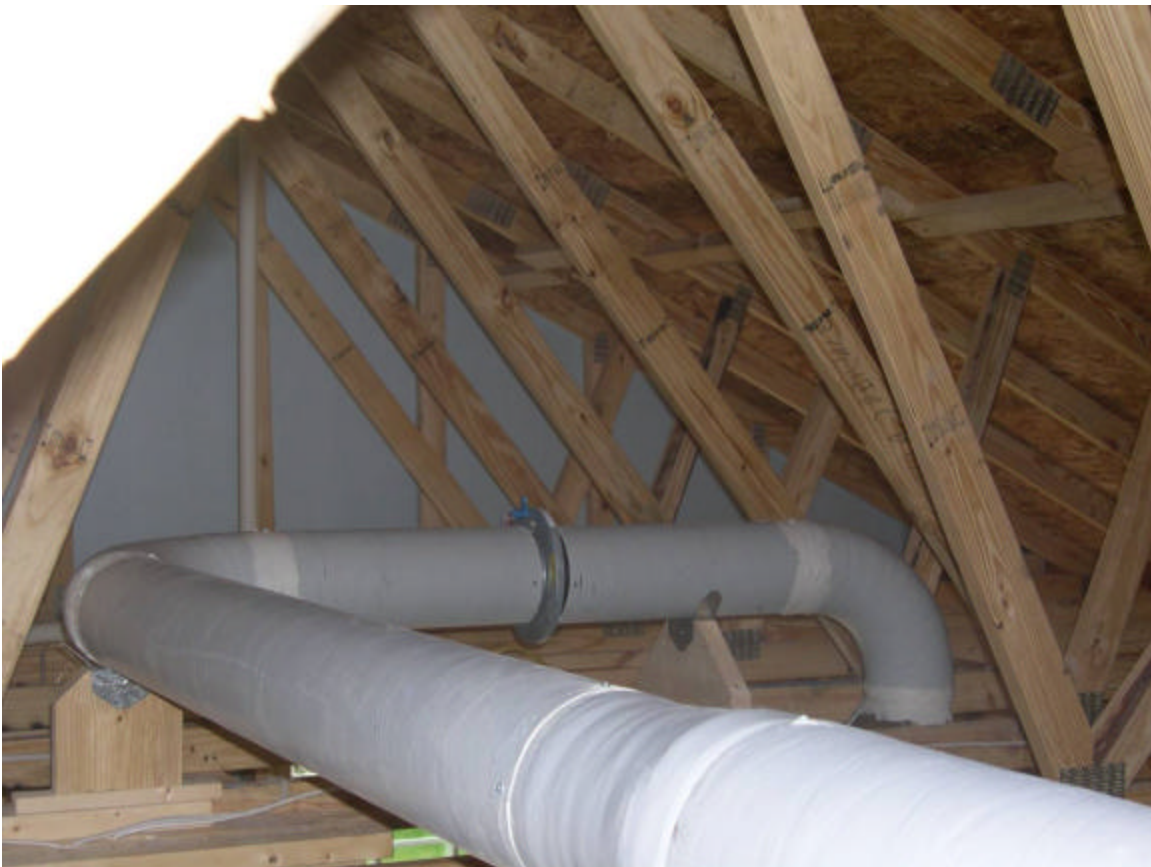
7" to 6" reduction with adjustable iris damper.
