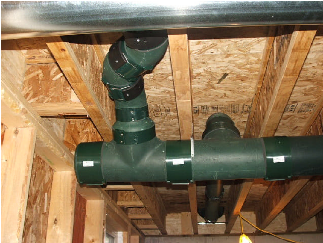
Spacing not always ideal for running between floor joists.
