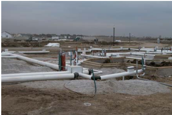
Figure 18 Underground PVC ductwork (extruded) for Cambridge Homes, Chicago's largest homebuilder.
