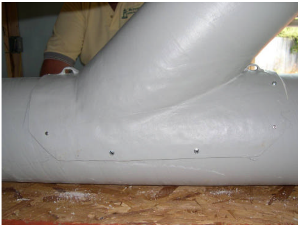
Saddle-type take off riveted to trunk.
