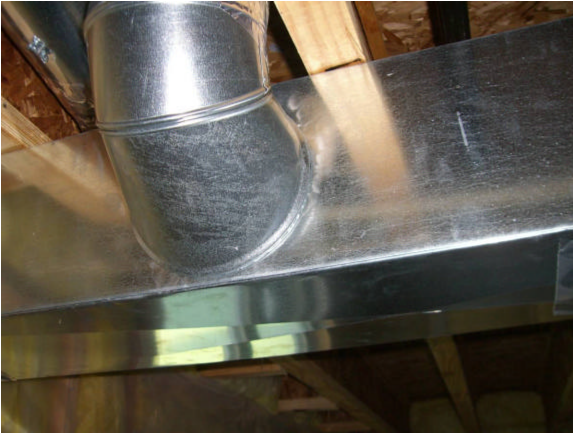
Smoke test indicating leakage at the take-off joint.
