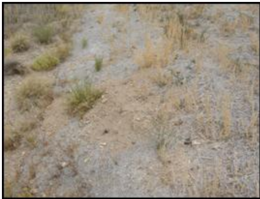
Figure 1. Small mammal burrows along the edge of the cover at CAU 407
