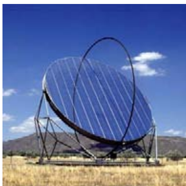
Figure S-4. The ASM 150-m 2 SM heliostat built by SBP/Steinmüller.
