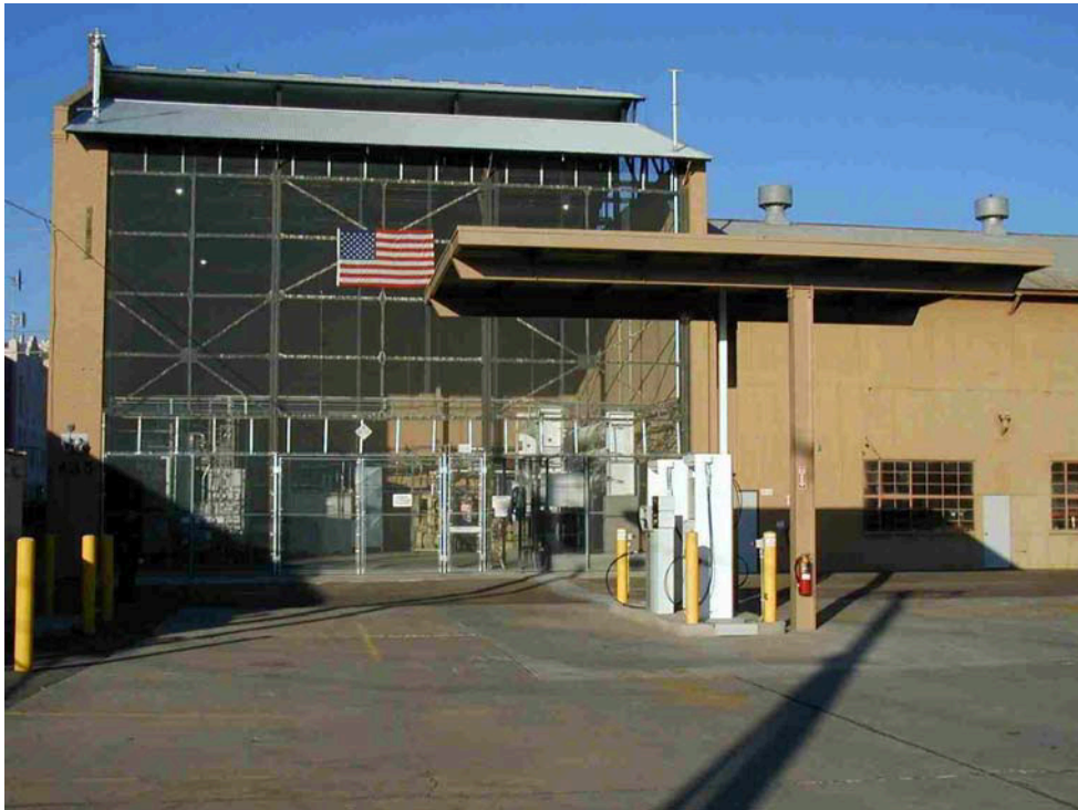
Figure 1. APS Alternative Fuel (Hydrogen) Pilot Plant, with the fueling dispensers in the foreground.
