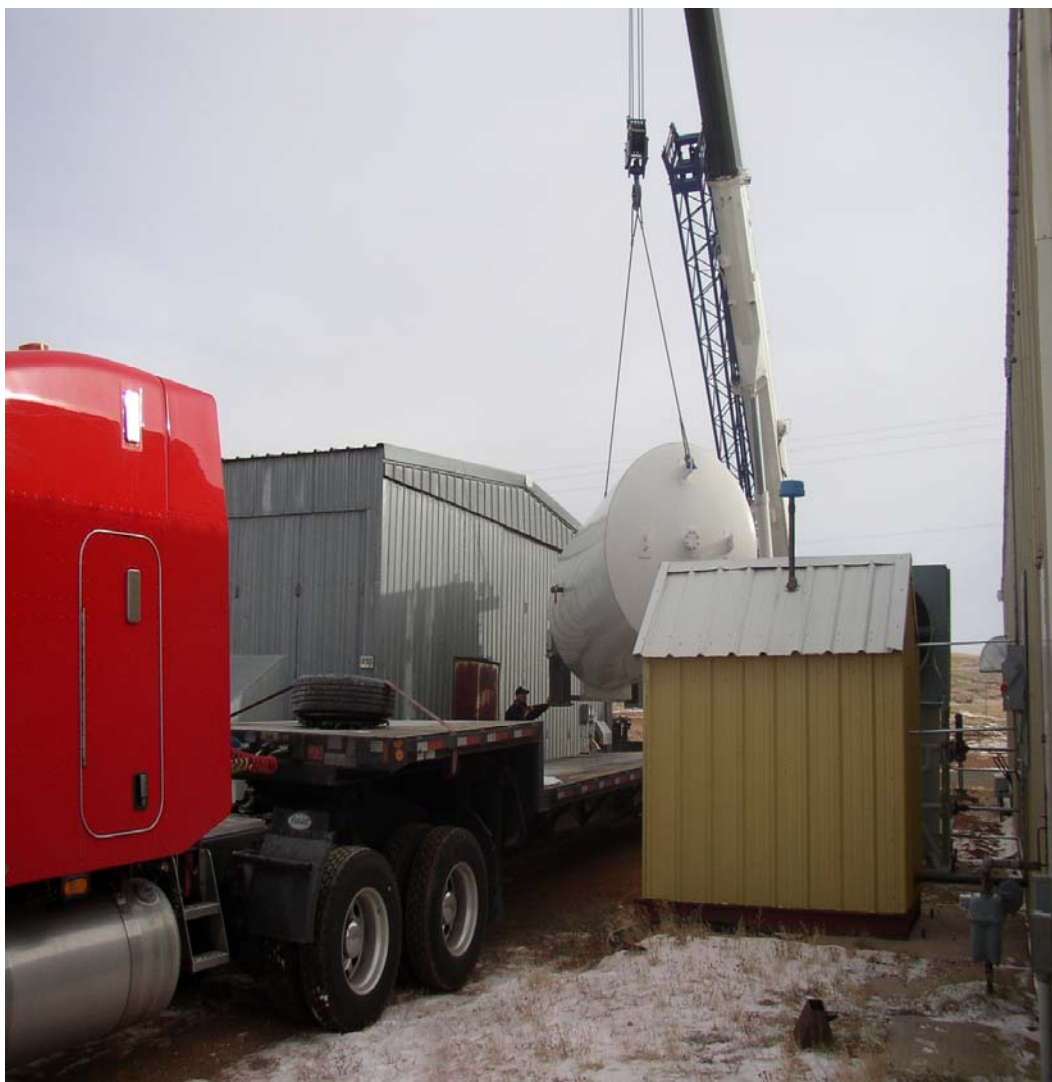
Figure 13. Installation of Carbon Dioxide Unit at WRI
