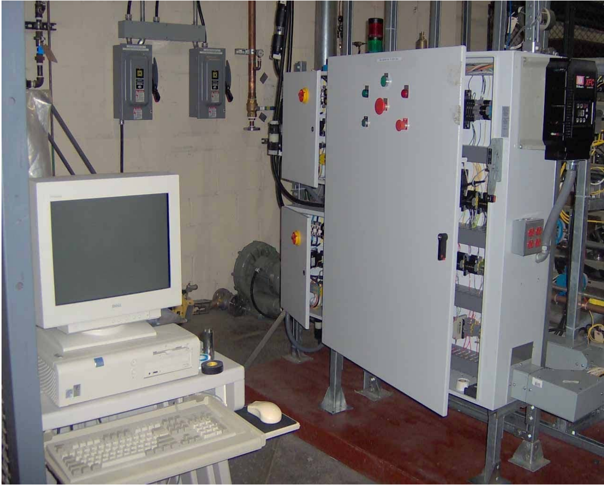
Figure 9. CAR PLC Controls Under Construction at BOC
