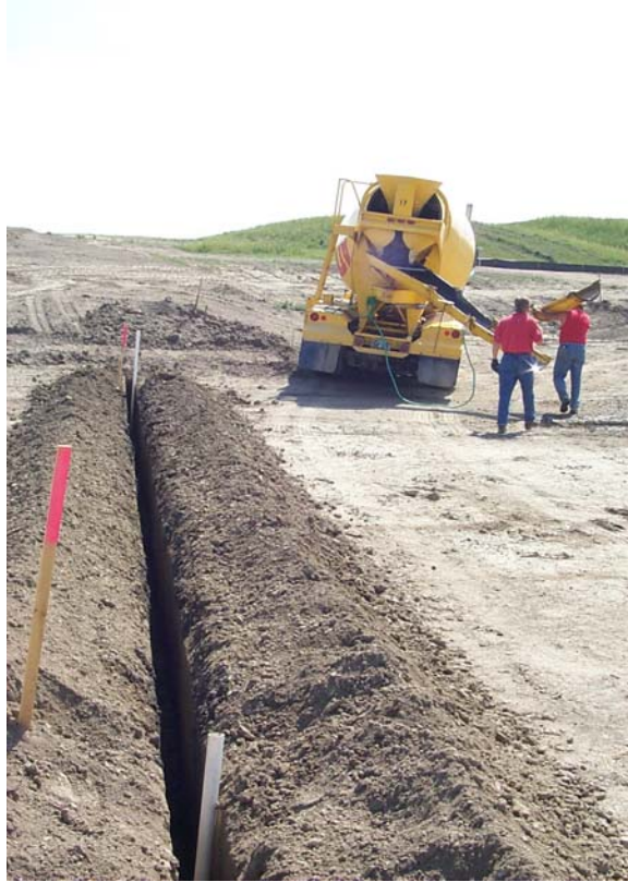
Figure 42. Excavated Utility Trench for Subdivision Development
