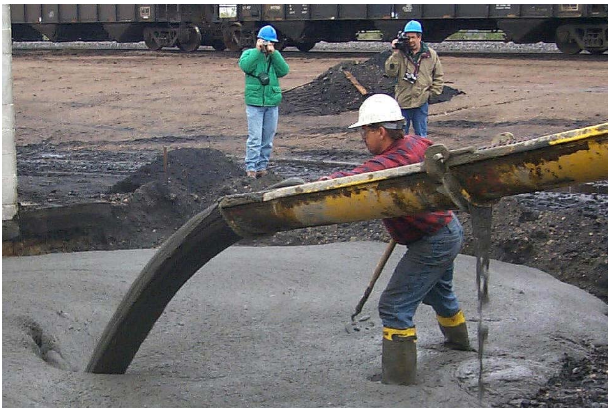
Figure 1. Photograph Showing the Flow Characteristics of MDU Flowable Fill Material
