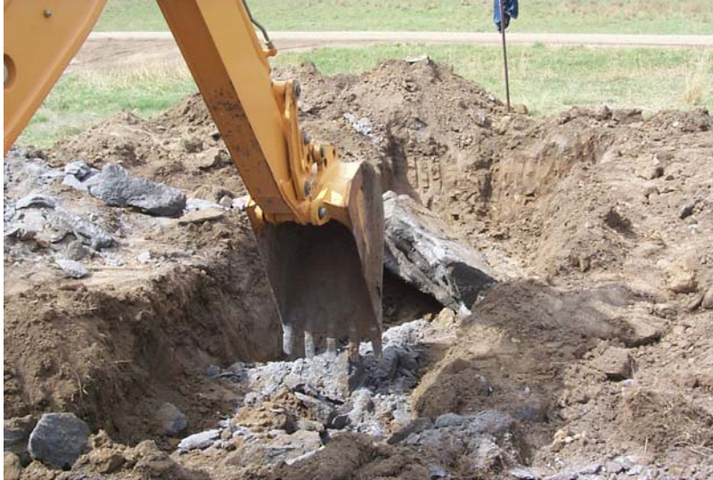
Figure 29. Excavation of the 30E Flowable Fill with a Toothed Bucket Backhoe
