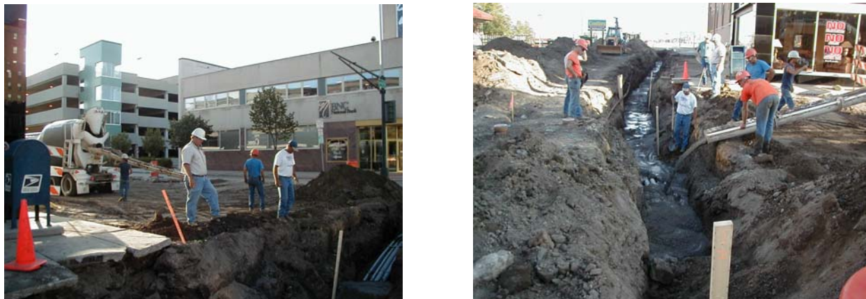
Figure 44. Photographs Showing the Placement of Ready-Fill as Part of the Main Street Repair Project in Bismarck, North Dakota
