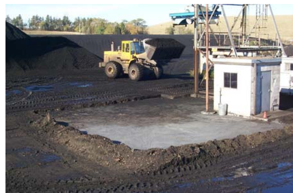
Figure 14. Condition of the Structural-Grade Flowable Fill Twenty Hours After Placement
