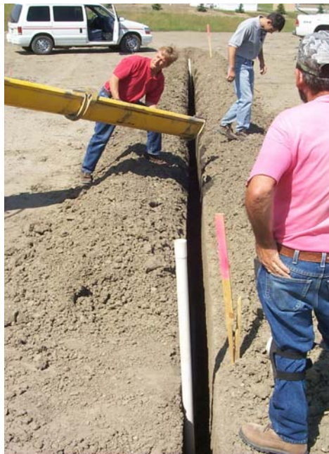
Figure 43. Placement of Ready-Fill for Utility Trench Fill
