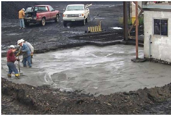
Figure 11. Placement of the Structural-Grade Fill
