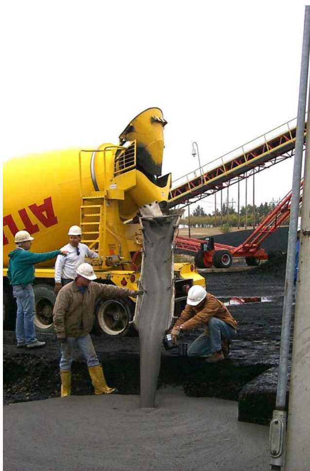
Figure 10. Placement of the Structural-Grade Fill
