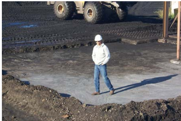
Figure 14. Condition of the Structural-Grade Flowable Fill Twenty Hours After Placement
