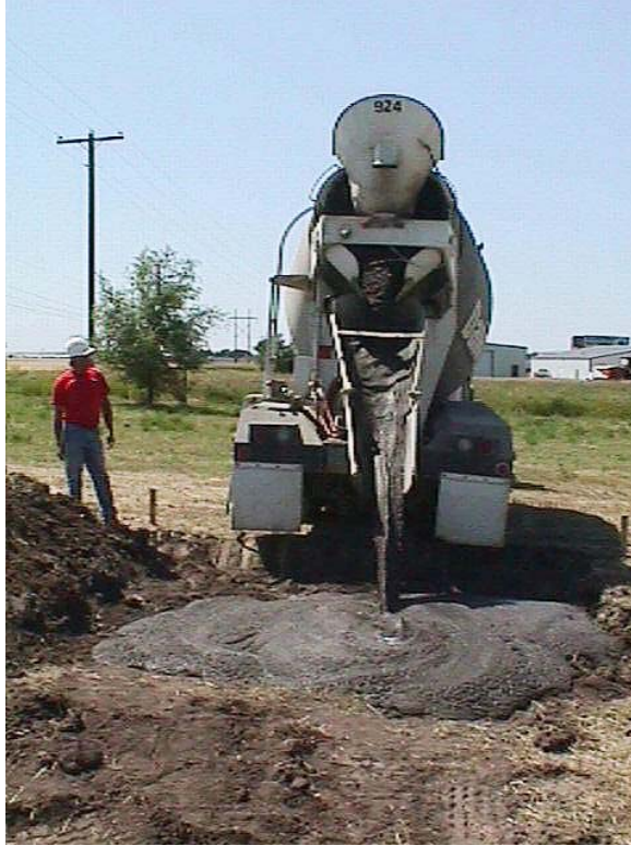
Figure 40. E-Grade Ready Fill Product Being Placed at Demonstration Site
