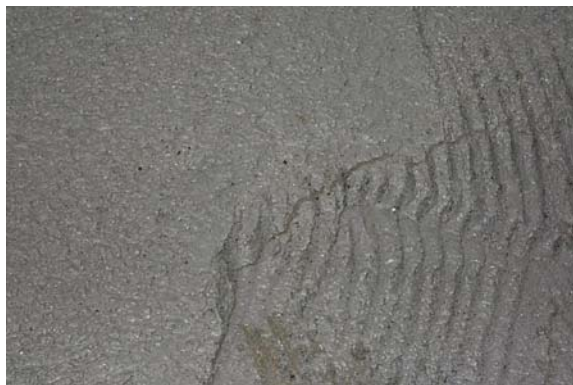
Figure 15. Photographs of the Surface Cracks that Developed on the Structural-Grade Fill
