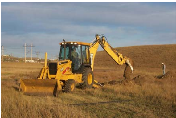
Figure 18. Construction of the Trenches for the 30E and 60E Demonstrations
