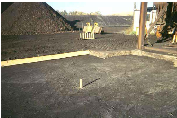
Figure 12. Setting of the Forms for the Concrete Pour
