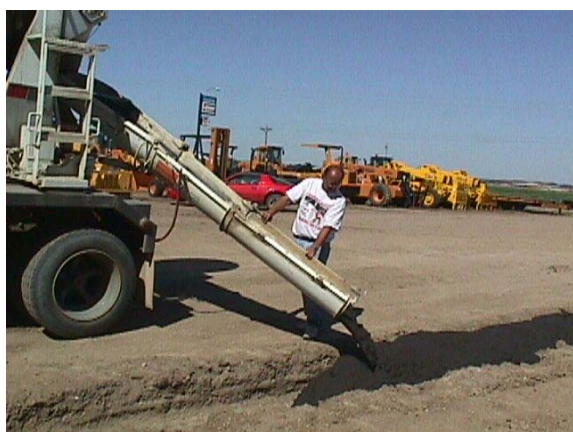
Figure 48. Placement of Ready-Fill at Krider Equipment Demonstration Site
