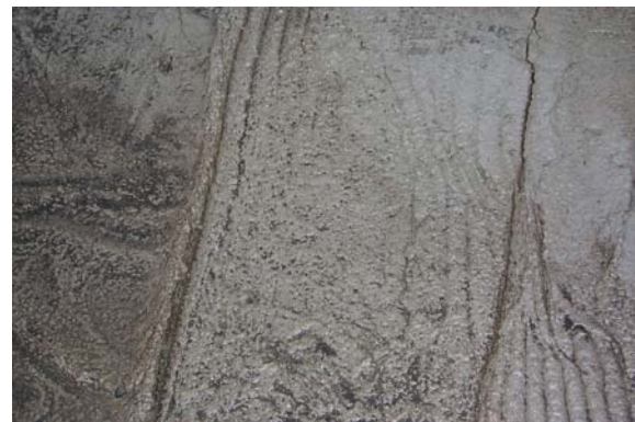
Figure 15. Photographs of the Surface Cracks that Developed on the Structural-Grade Fill
