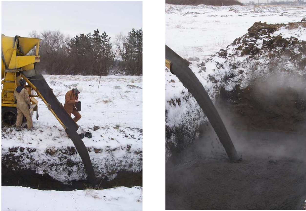
Figure 23. Photographs of the Placement of the 10E200 Flowable Fill Material at the Demonstration Site
