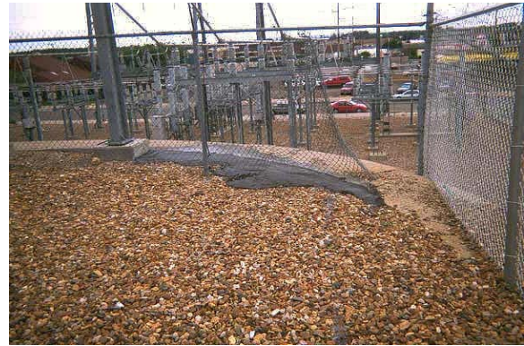
Figure 52. Poured Ready-Fill Repair at the MDU Sweet Avenue Substation
