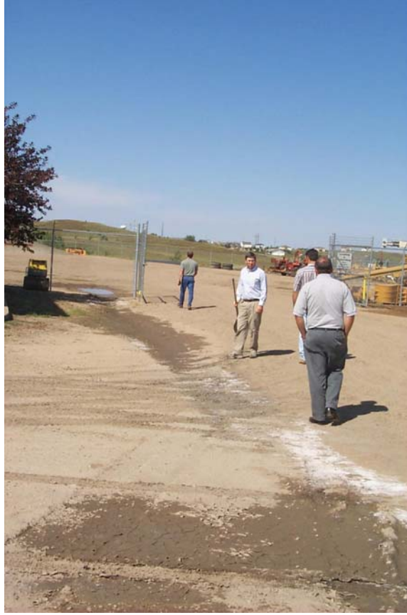
Figure 50. Monitoring the Storm Water Drainage Ditch Made From Ready-Fill at Krider Equipment
