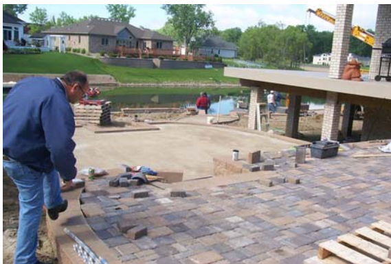
Figure 53. Photographs of the Use of Ready-Fill Product for Construction of a Bricked Residential Patio
