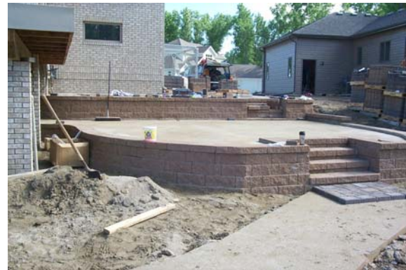
Figure 53. Photographs of the Use of Ready-Fill Product for Construction of a Bricked Residential Patio
