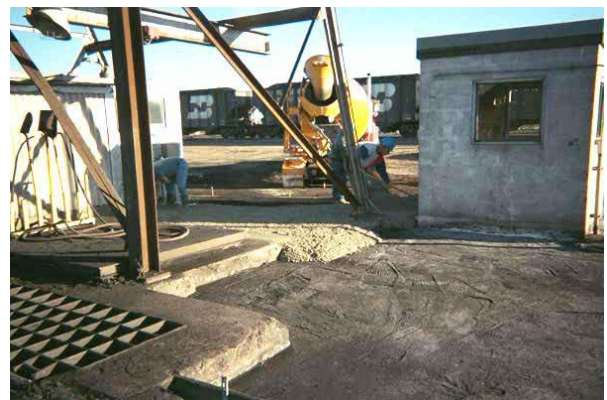
Figure 13. Concrete Pour at Structural-Grade Flowable Fill Demonstration Site
