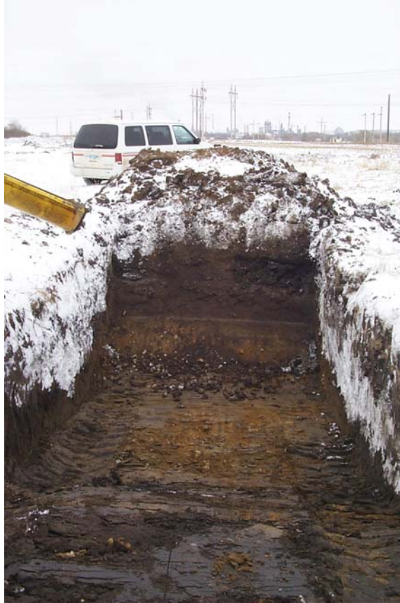
Figure 20. Construction of the Trench for the E200 Fill Demonstration
