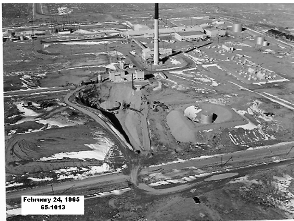
Figure 1-15. Photograph of Bin Set 2 during construction showing vault foundation and southern portion of the CPP-93 Trench (view looking west).
