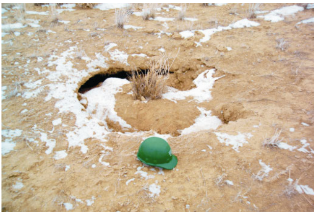
Figure 16. Subsidence in CFA Landfill III. (P-1216-06.JPG)
