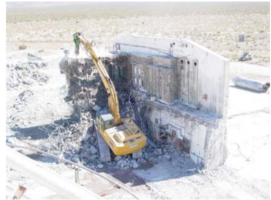
Figure 5. Mechanical Demolition
