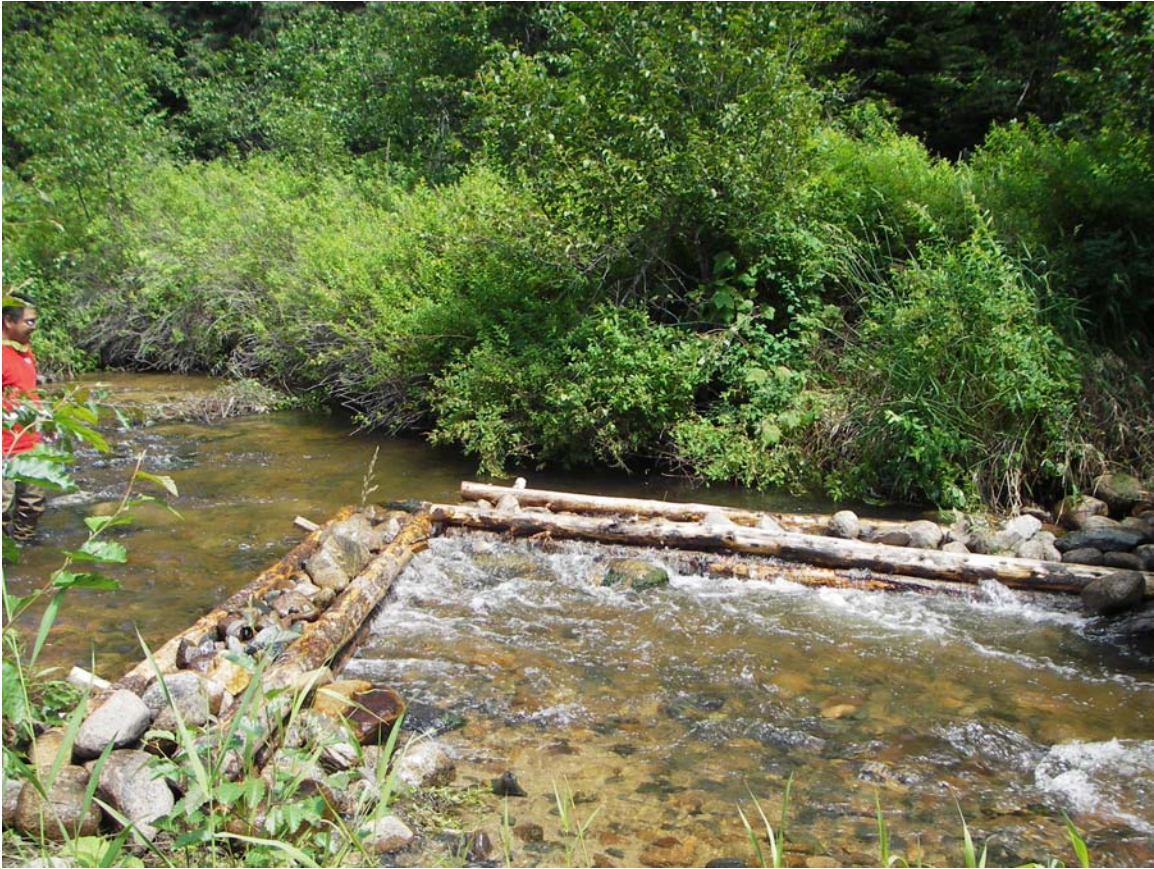
Figure 52. Engineered LWD piece constructed in 2005 in East Branch LeClerc Creek.
