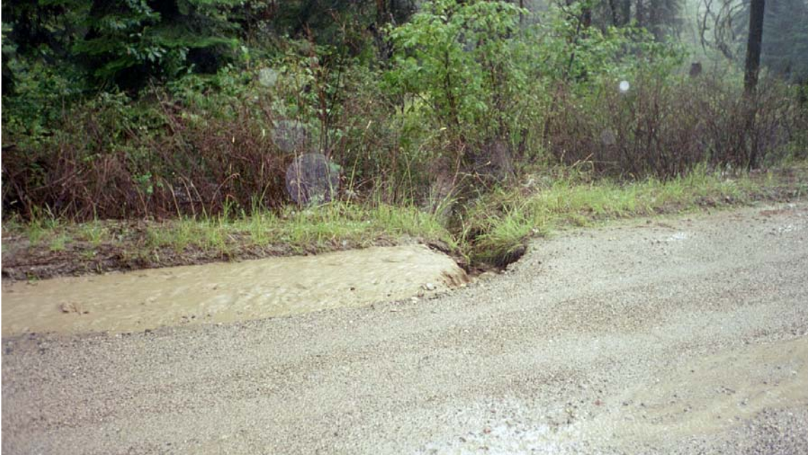
Figure 22. Forest Service Road 1934 contributing fine sediment to the stream channel.
