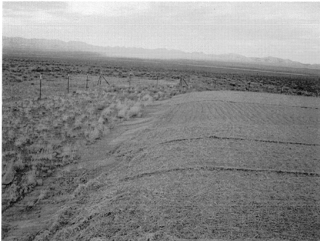
Photograph 24: CAU 407, Erosion Blanket, 12/01/2004
