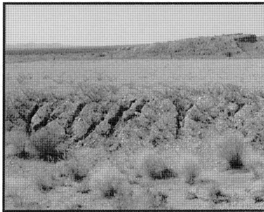
Figure 3. June 4, 2004. Erosion gullies along northern edge of the soil cap at CAU 407.
