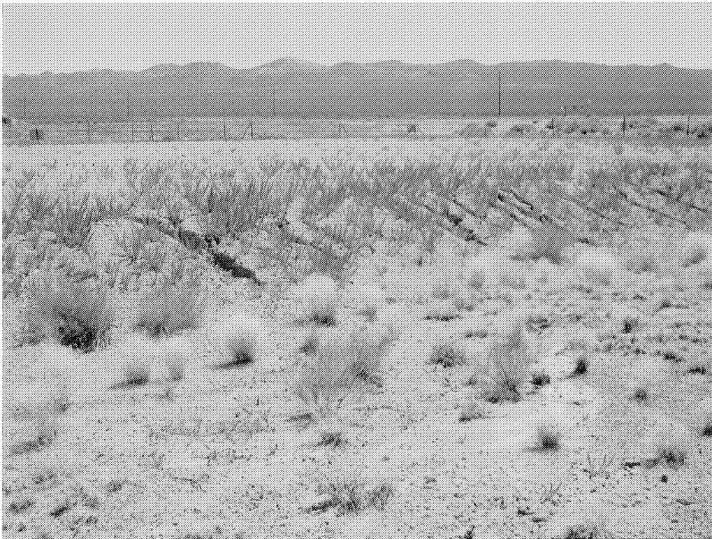
Photograph 17, CAU 407, Erosion rills on the east side of the cover, 07/07/2004
