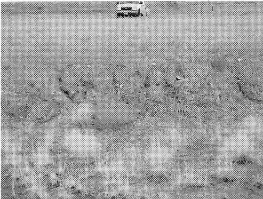
Photograph 18, CAU 407, Erosion rills on the east side of the cover, 11/09/2004
