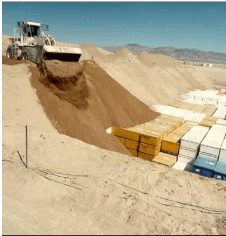
Figure 4-2 Emplacement of Backfill Over Waste Containers
