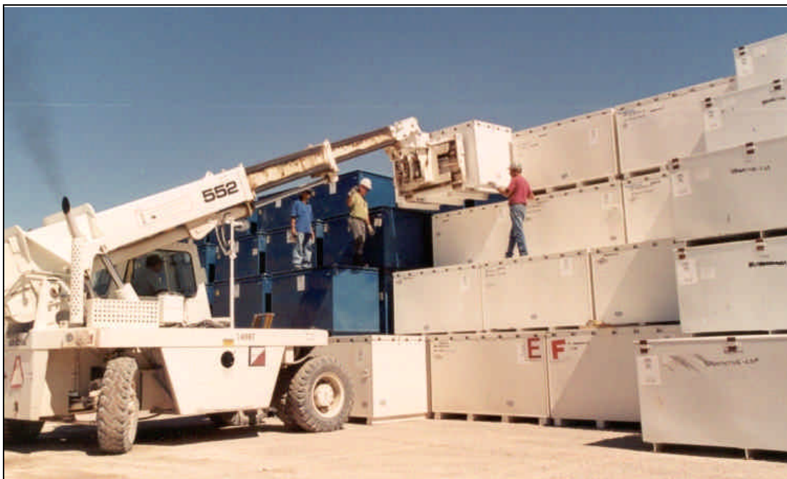
Figure 4-1 Waste Container Emplacement in a Typical Pit at the Area 5 Radioactive Waste Management Site
